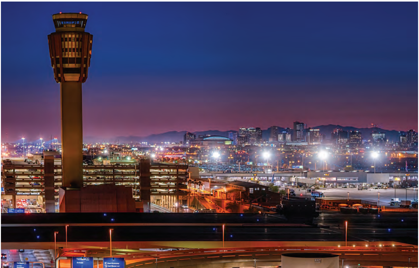
The U.S. DOT Volpe Center team designed a sprinkler system replacement and a fire/life safety upgrade package for the ATCT at Phoenix Sky Harbor International Airport. Source: Adobe Stock / brent coulter
