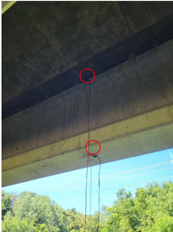
(a) Strain gauges on top and bottom flange
