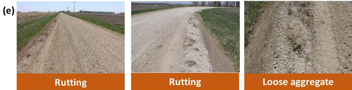
Figure 114. Representative distresses of each road section: (a) K45, (b) E60 (AC-surfaced pavement section), (c) E60 (PCC-surfaced pavement section), (d) Filbert Avenue, and (e) 295th Street
