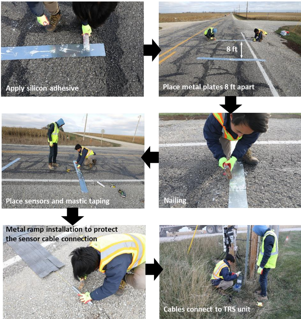
Figure 118. Installation procedures of a P-WIM system
