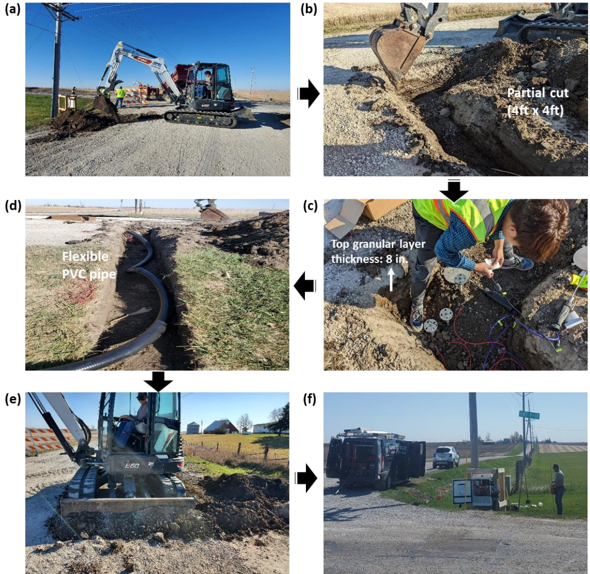
Figure 95. Steps of the sensor installation: (a) trench cutting for the PVC pipe route, (b) excavating the designated area of the road, (c) installing the sensors, (d) protecting sensor cables through flexible PVC pipe, (e) backfilling and compacting the damaged road, and (f) activating the external power supply
