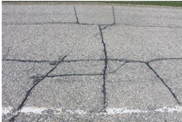
Transverse crack
