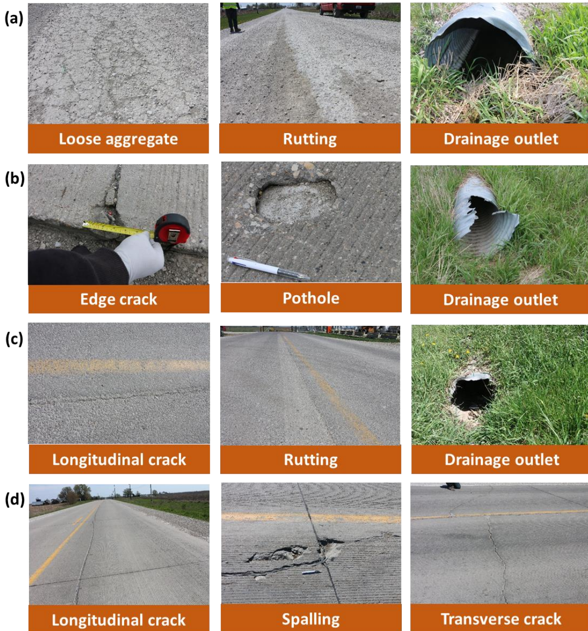
Figure 109. Representative distresses and features of each road section: (a) Osage Street, (b) North Osage Street, (c) Rea Road, and (d) Cherry Street
