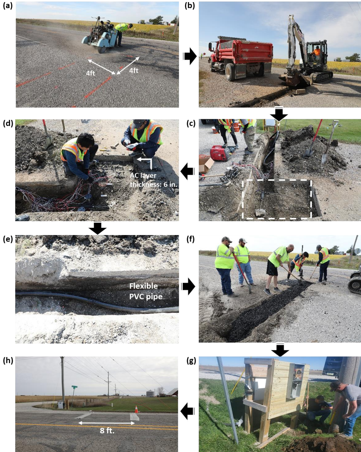
Figure 86. Steps of the data acquisition system installation: (a) pre-cutting a portion of the road, (b) trench cutting for the PVC pipe route, (c) excavating the designated portion of the road, (d) installing the sensors, (e) protecting sensor cables through flexible PVC pipe, (f) repairing the damaged road, (g) connecting the external power supply, and (h) installing P-WIM system
