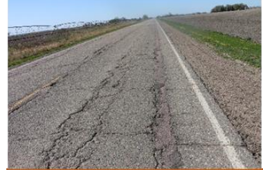
Block crack
