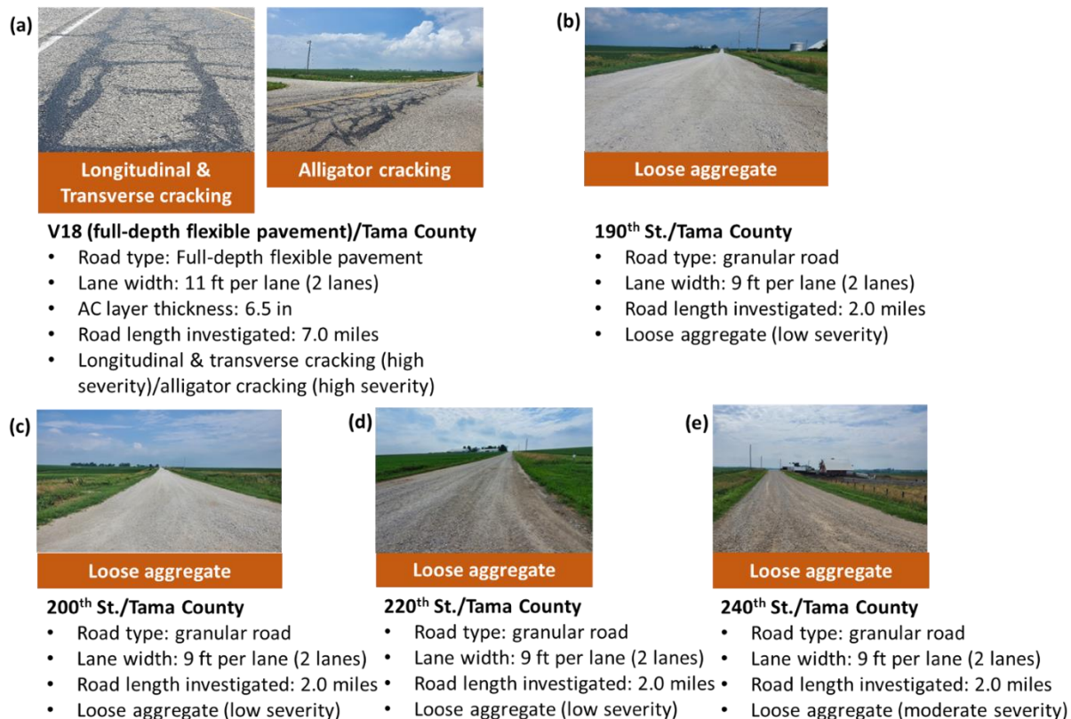
Figure 65. Summary of the forensic investigation results conducted in Tama County at (a) V18 and (b) 190 th , (c) 200 th , (d) 220 th , and (e) 240 th streets
