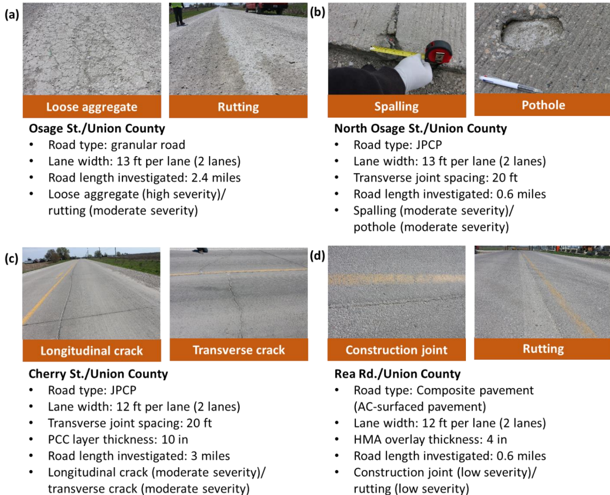
Figure 59. Summary of the forensic investigation results conducted in Union County at (a) Osage Street, (b) North Osage Street, (c) Cherry Street, and (d) Rea Road
