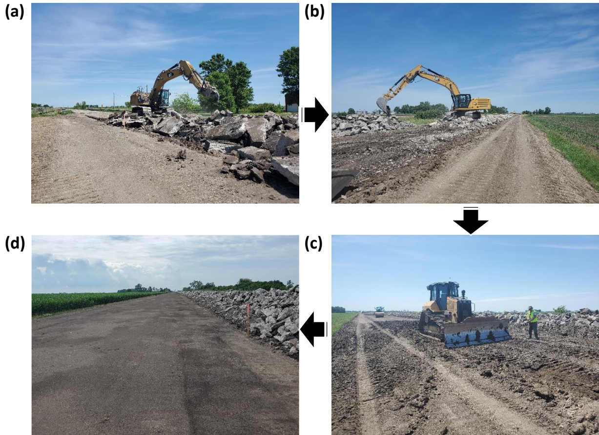
Figure 73. JPCP reconstruction process: (a) excavation of existing composite pavement, (b) removal and (c) gradation, to (d) expose the subgrade soil
