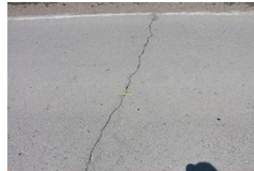
Transverse crack
