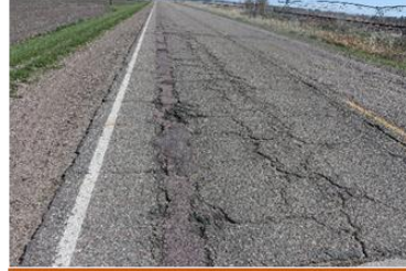
Transverse crack
