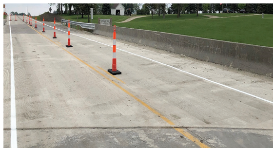
LMC-VE overlay on the IA 15 bridge over Black Cat Creek (May 20, 2023)
