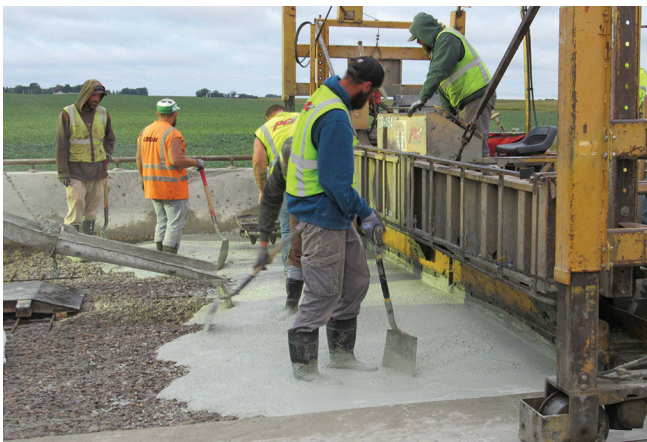
Placement of LMC-VE overlay material
