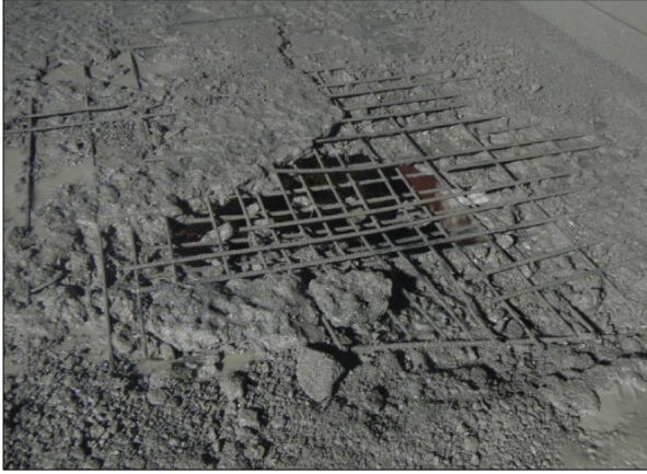
(a) Punch-through in deck, post hydrodemolition
