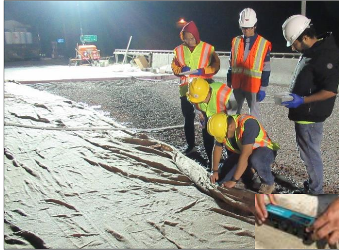
(a) On-site SR measurements
