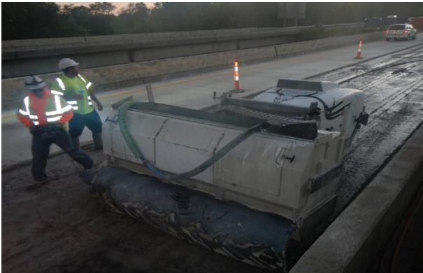
(c) Hydrodemolition to remove distressed concrete
