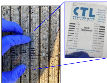
(c) Crack comparator used for crack width measurement
