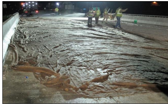
(d) Wet burlap kept for 4 hours of wet curing
