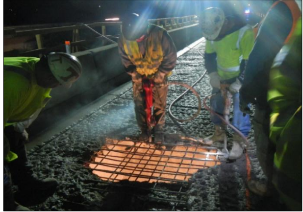
(b) Repairing punch-through by jackhammering to remove loose concrete
