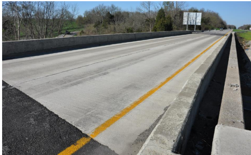
(e) Finished bridge deck
