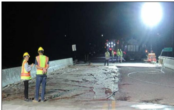
(e) Overlay cast on half of the deck surface
