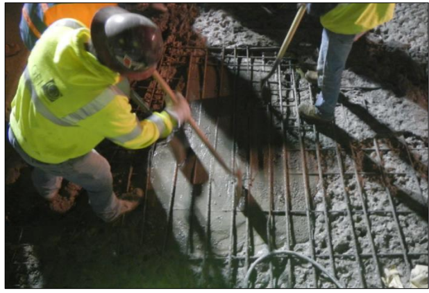
(d) Patching material being applied to fill the punch-through
