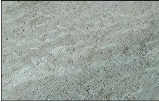
(a) Overlay surface after wet burlap removal
