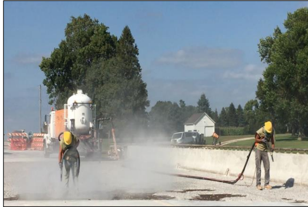
(a) Overview of sand-blasting operation
