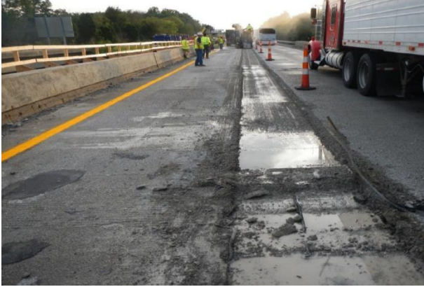
(a) Bridge deck after surface milling
