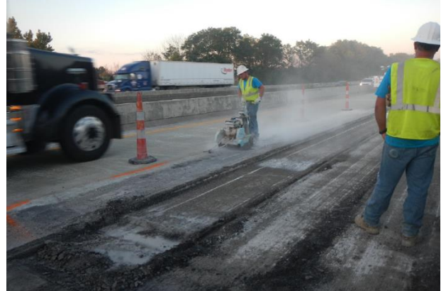
(b) Vertical perimeter of overlay work being sawed
