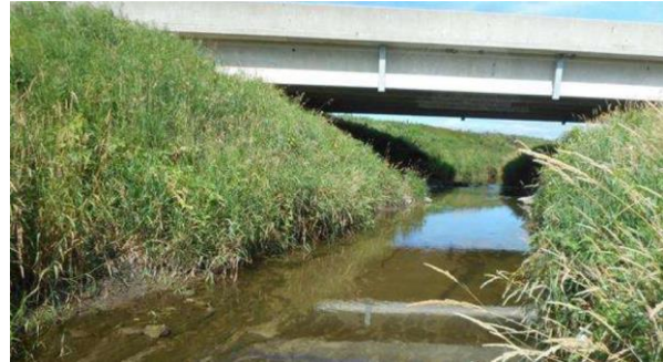
(b) Side profile of the bridge
