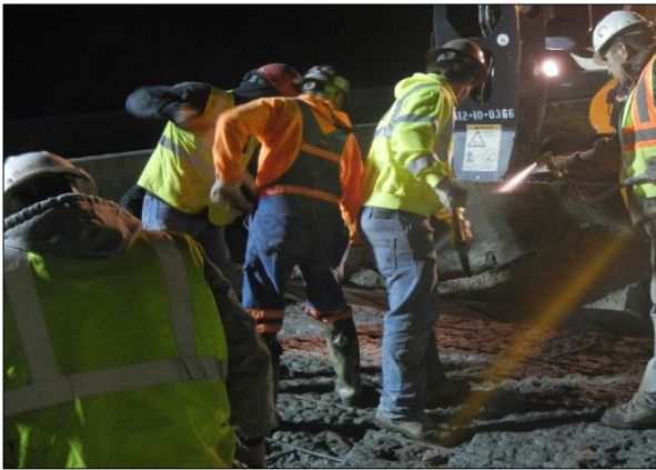
(c) Duracal patching compound being mixed to fix the punch-through
