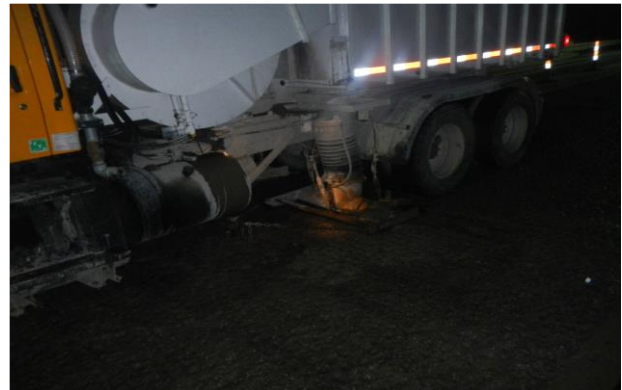
(d) Vacuum truck cleaning concrete debris from the deck after hydrodemolition
