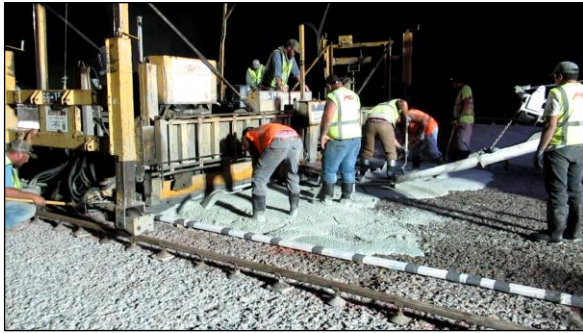
(a) Overview of the overlay casting operation
