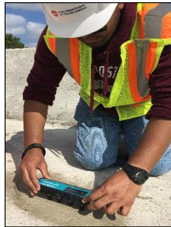
(a) SR measurement on the overlay surface
