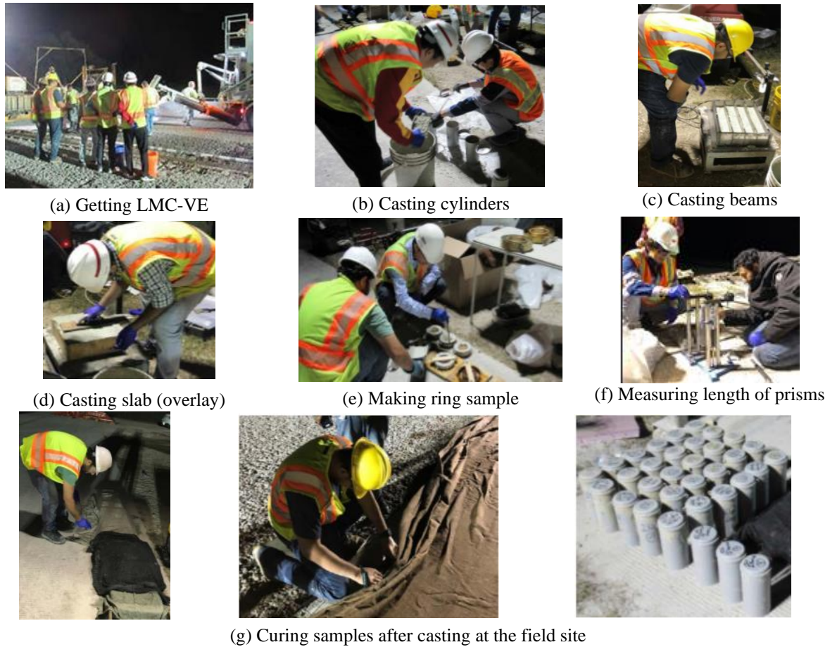
Figure 3.17. Casting test specimens during overlay construction
