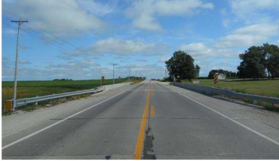
(a) Old deck surface
