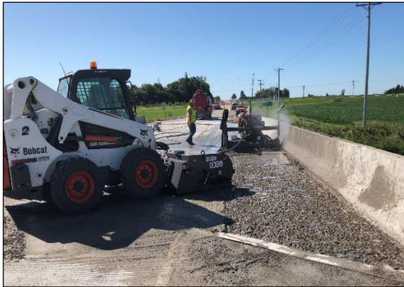
(a) Overview of the hydrodemolition operation
