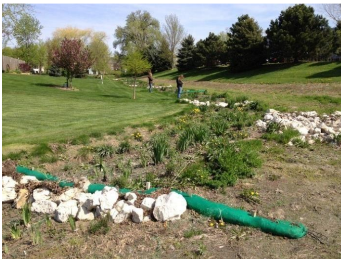
Figure 2.8. Bioswale (Iowa stormwater management, 2017)
