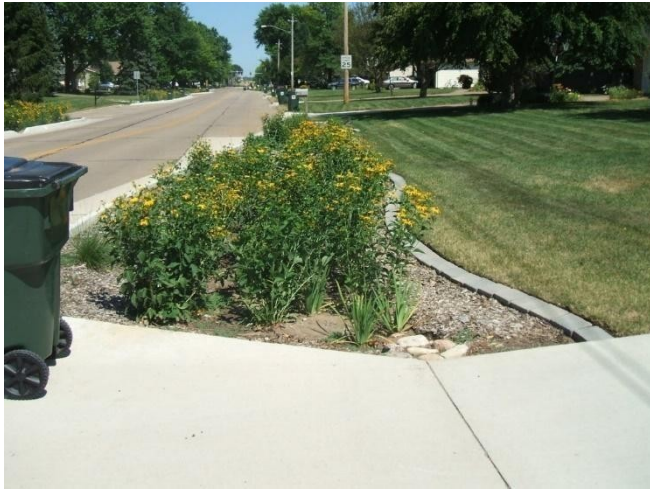
Figure 2.7. Bioswale adjacent to a roadside (Iowa stormwater management, 2017)
