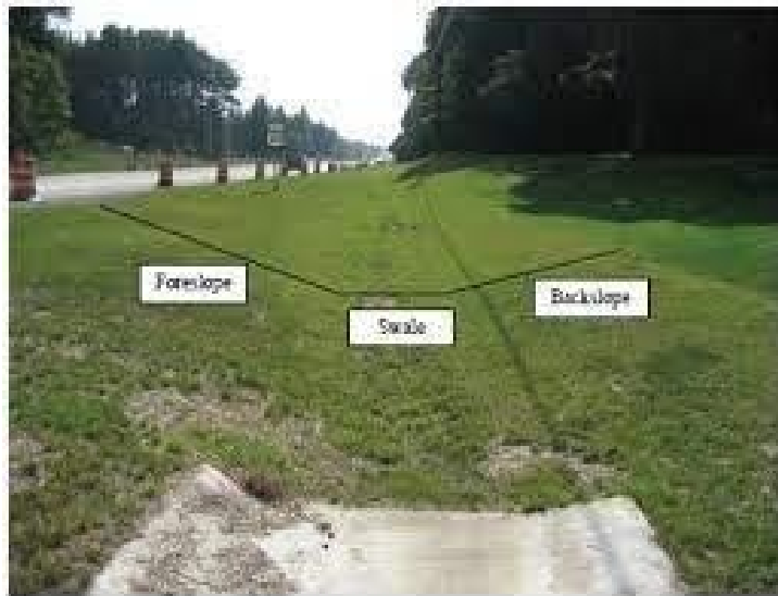
Figure 2.1. Biofiltration system with vegetated foreslope, backslope, and swale (Mitchell et al., 2010).
