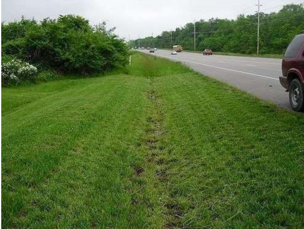
Figure 1.1 Biofiltration system along a highway in Montana (Flexamat, 2002)
