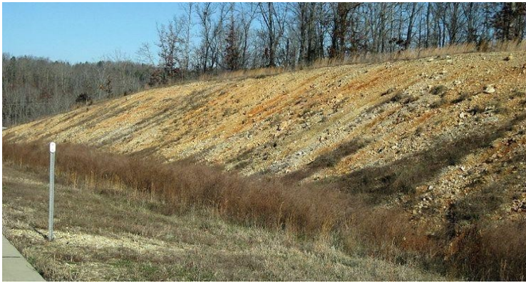
Figure 2.3. Bioslope at Crow Wing County, Minnesota Stormwater Manual (2018)
