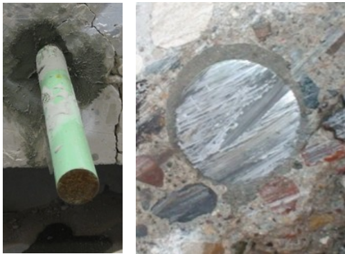
Adhesive Sample Test Hole #41 – Non-Shrink Grout
