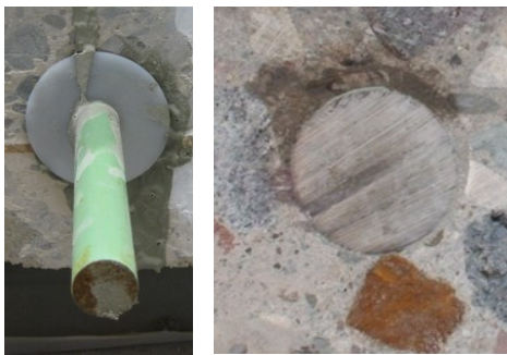
Adhesive Sample Test Hole #36 – Non-Shrink Grout
