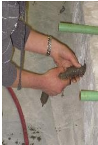
Figure 10. Insertion of Saturated Grout Capsule into Pre-Drilled Hole
