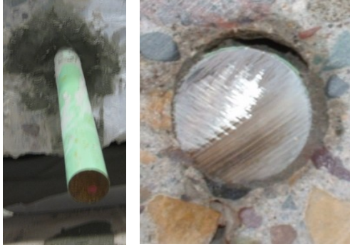
Adhesive Sample Test Hole #35 – Non-Shrink Grout
