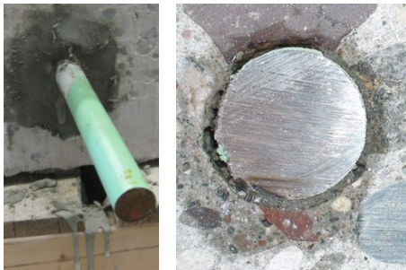
Adhesive Sample Test Hole #31 – Non-Shrink Grout
