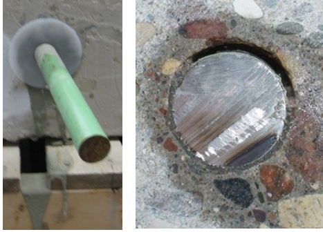
Adhesive Sample Test Hole #32 – Non-Shrink Grout
