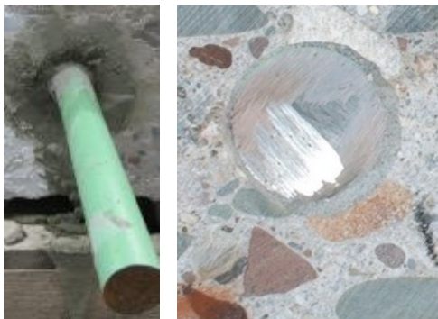
Adhesive Sample Test Hole #38 – Non-Shrink Grout
