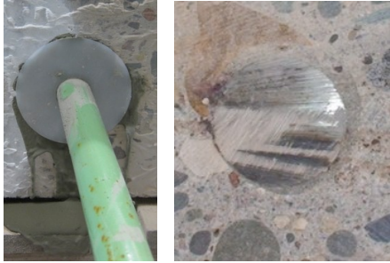
Adhesive Sample Test Hole #39 – Non-Shrink Grout
