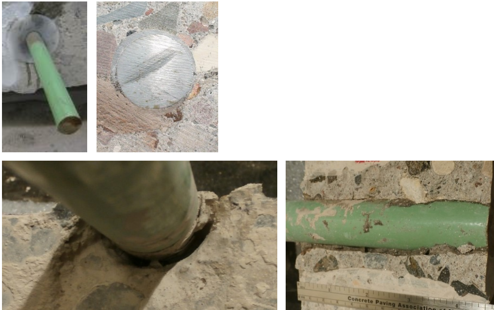
Adhesive Sample Test Hole #25 - Cementitious Anchoring Capsule Grout
