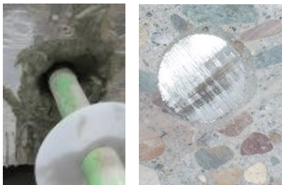
Adhesive Sample Test Hole #37 – Non-Shrink Grout
