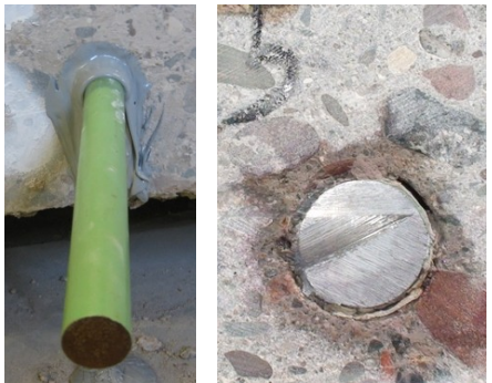
Adhesive Sample Test Hole #5 - Double Dip Two Part Epoxy / Hand Mixed
