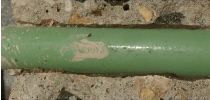
Adhesive Sample Test Hole #30 - Cementitious Anchoring Capsule Grout
