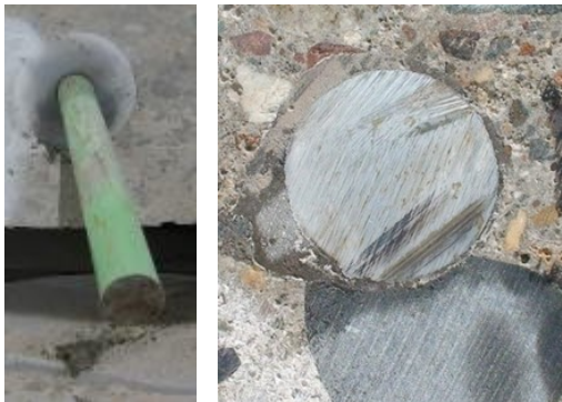
Adhesive Sample Test Hole #27 - Cementitious Anchoring Capsule Grout
