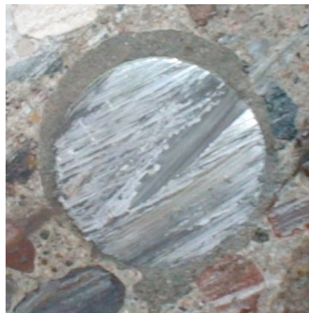
Figure 18. Dowel Hole Location 41 - Significant Reflection with No Voids Present
