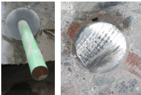
Adhesive Sample Test Hole #34 – Non-Shrink Grout
