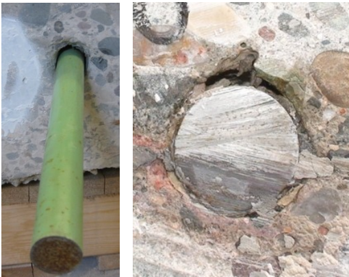
Adhesive Sample Test Hole #10 - Epoxy filled hole
