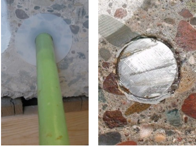
Adhesive Sample Test Hole #9 - Epoxy filled hole
