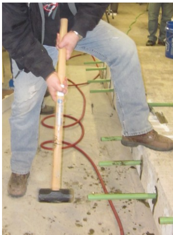
Figure 11. Insertion of Dowel Bar into Pre-Drilled Hole
