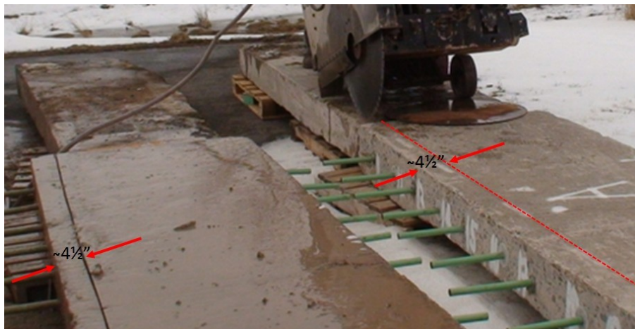
Figure 5. Preparing to cut the second Concrete Panel at 4.5" from panel face
