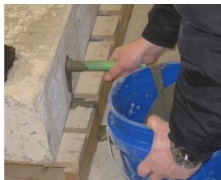
Figure 8. Grout - Dip Method Insertion
