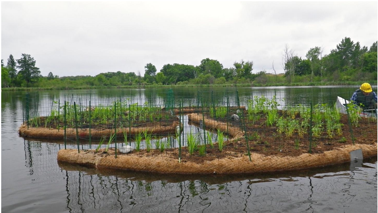
Figure 2-7: Floating treatment wetland (recently constructed) at the Tamarack Nature Center in White Bear Lake, MN. Photo: https://midwestfloatingisland.com/
