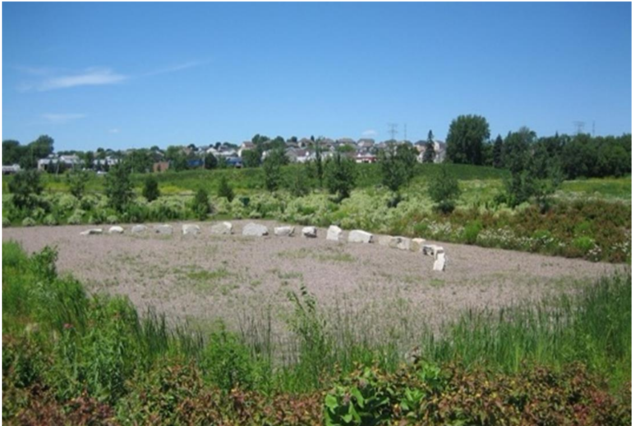
Figure 5-6: Beam Avenue iron enhanced sand filter (Ramsey Washington Metro Watershed District). Flow enters the basin, filters through pea gravel on the surface, and iron enhanced sand below the pea gravel, and finally into pea gravel that allows the flow to be exported by drain tiles. Photo: Andy Erickson.
