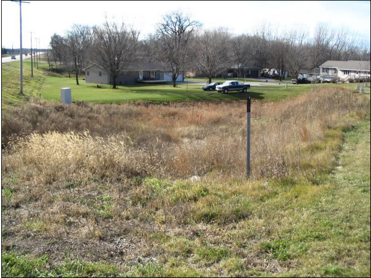
Figure 6-3: Infiltration basin with natural grass covering. Photo: John Gulliver.
