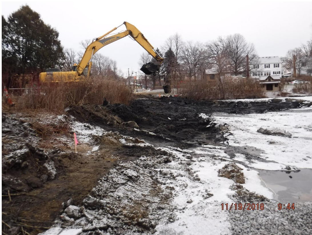
Figure 2-6: Water levels in a wet pond are drawn down to facilitate dredging with a backhoe. Photo: Noah Czech, City of St. Cloud, MN.
