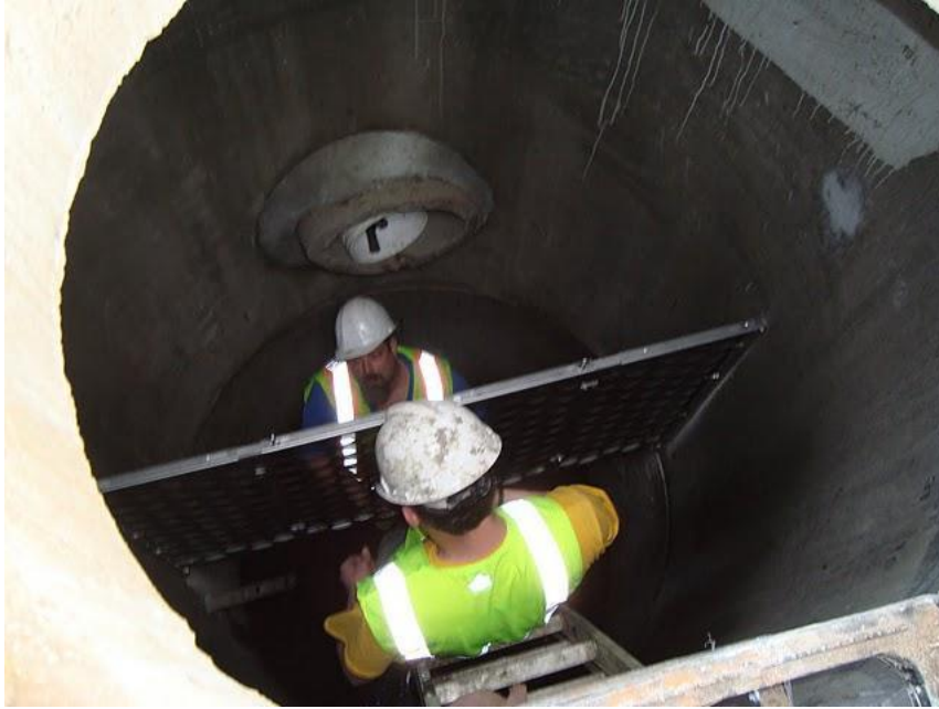
Figure 3-3: SAFL baffle inserted into an existing sump catch basin. Photo: Upstream Technologies.
