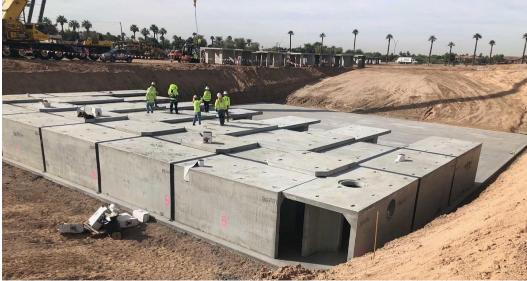
Figure 3-4: Installation of a wet vault in Litchfield Park, AZ. Photo: Contech Engineered Solutions.
