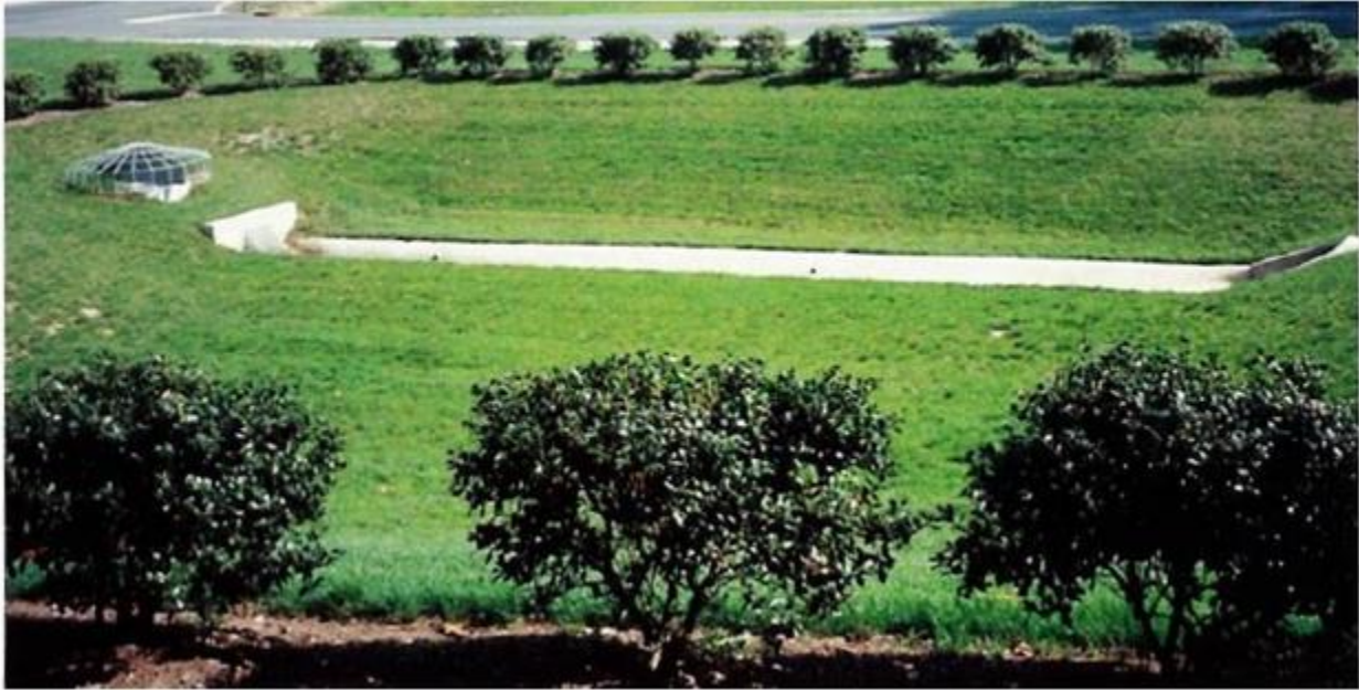
Figure 2-4: Example of a dry detention pond (MPCA 2023).
