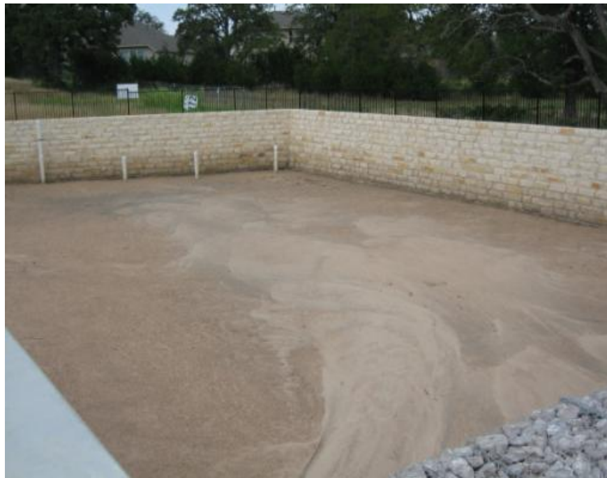
Figure 5-1: Typical surface sand filter in Austin, Texas. Photo: Andy Erickson.
