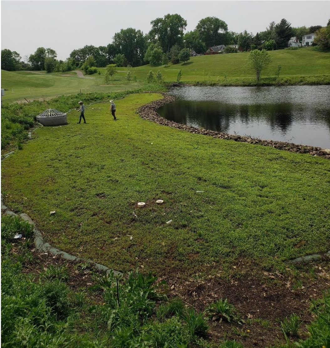
Figure 5-7: Como Golf Course Pond IESF in St Paul (Capitol Region Watershed District). Pond, filter covered with vegetation, and grate covered overflow structure are shown. The IESF has two drain tiles, both discharging to the same structure. Photo: Peter Weiss.
