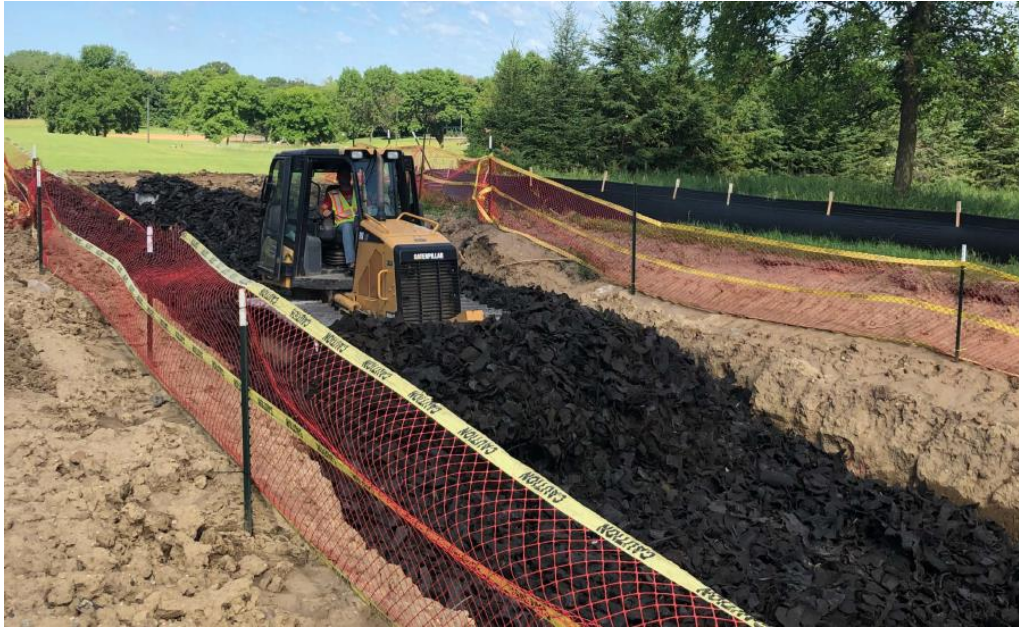
Figure 3-5: Installation of tire derived aggregate as an underground storage and sedimentation chamber. Photo: TDA Manufacturing
