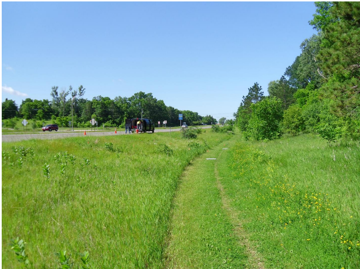
Figure 6-4: Bioswale to accept road runoff, infiltrate stormwater, convey stormwater and improve the water quality of stormwater. Photo: John Gulliver
