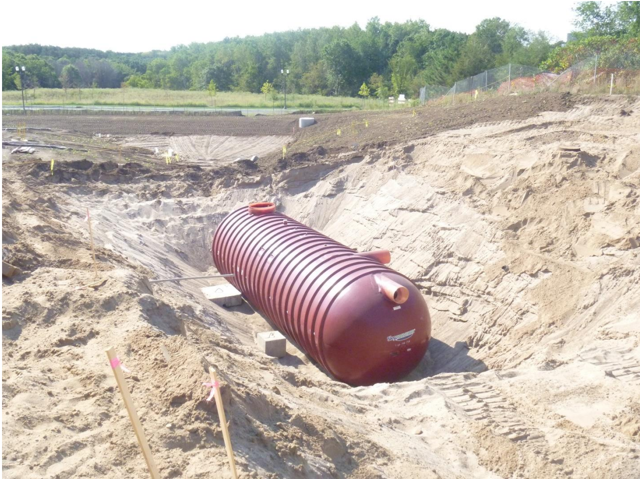
Figure 8-2: Photo of tank for harvest and use system. Photo: City of Cottage Grove.
