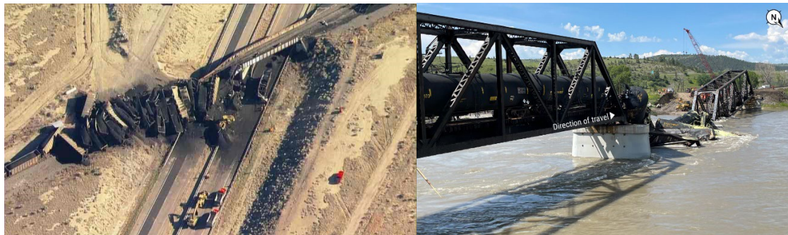
Figure 1.1 Two significant derailment failures: Left: 30 BNSF rail cars hauling coal near Pueblo, Colorado, derailed on October 15, 2023, causing extensive damage and one death on I-25 below the bridge (photo courtesy of KVDR); right: 16 rail cars, 15 of which had hazardous material, derailed on June 24, 2023, at Reed Point, Stillwater County, Montana (photo NTSB). In the former case, the tracks had been inspected on the day of the accident.
