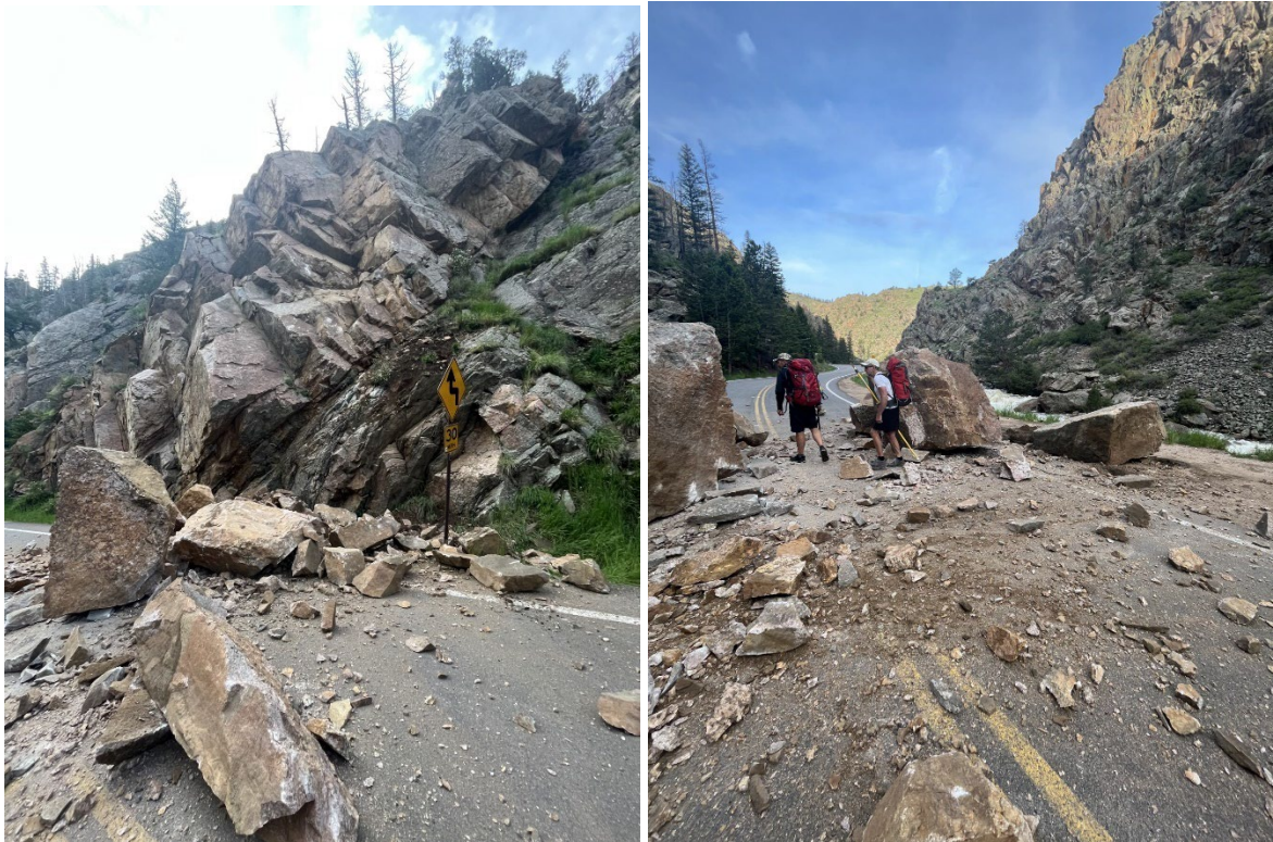
Figure 3.1 Rockfall damage on Highway 14 on June 9, 2023, at 6 AM. The PI and colleagues (right) were on scene to investigate the level of damage and attempt to image the resulting starting and final position of the rockfall. The highway was closed for about four hours, but after an incredible response by CDOT was shortly reopened despite significant damage to the surrounding asphalt.
