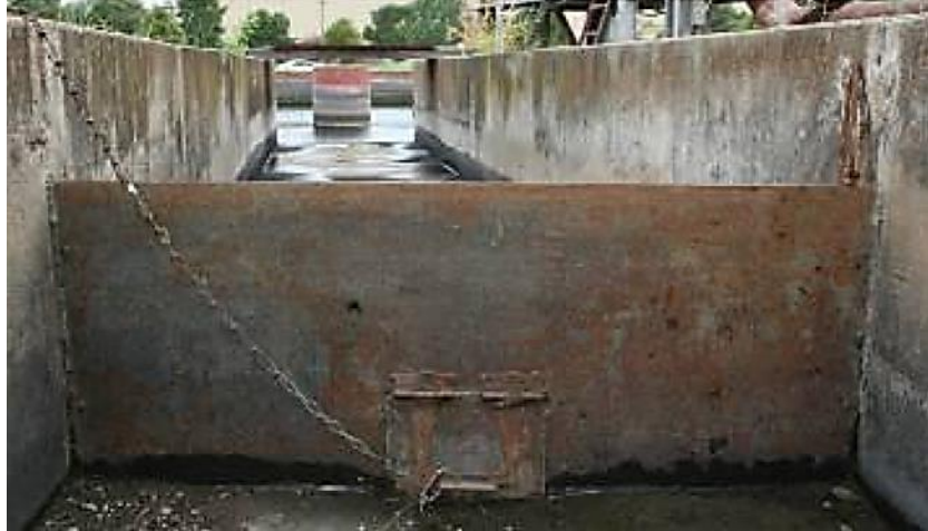
Figure 4.8. Discharge Weir and Orifice Gate (15).
