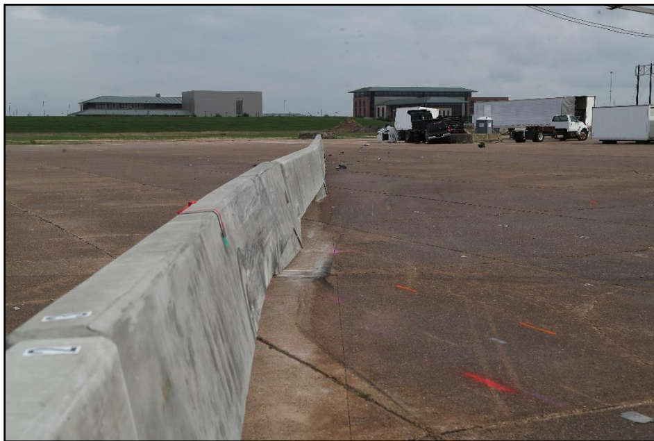
Figure 10.5. Large-Scupper Portable Concrete Barrier after Test at Impact Location for Test 440873-01-2.
