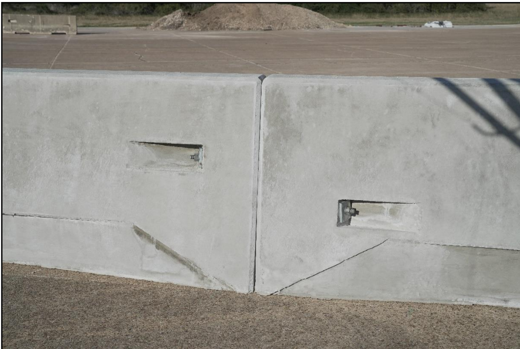
Figure 6.3. Large-Scupper Portable Concrete Barrier at the Joint of Barriers 3 and 4 prior to Testing.
