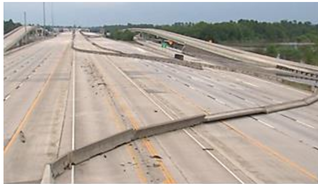
a. Portable concrete median barrier in Humble, Texas.
