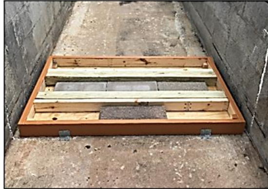
Figure 4.4. Support Base Design and Installation (15).
