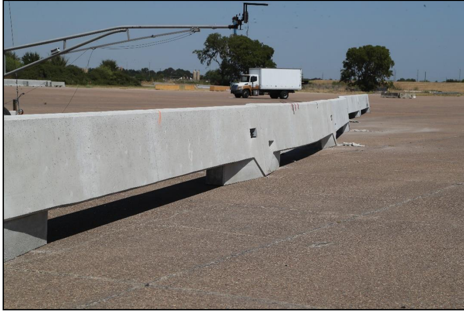
Figure 11.6. Large-Scupper Portable Concrete Barrier at the Field Side after Test 440873-01-3.
