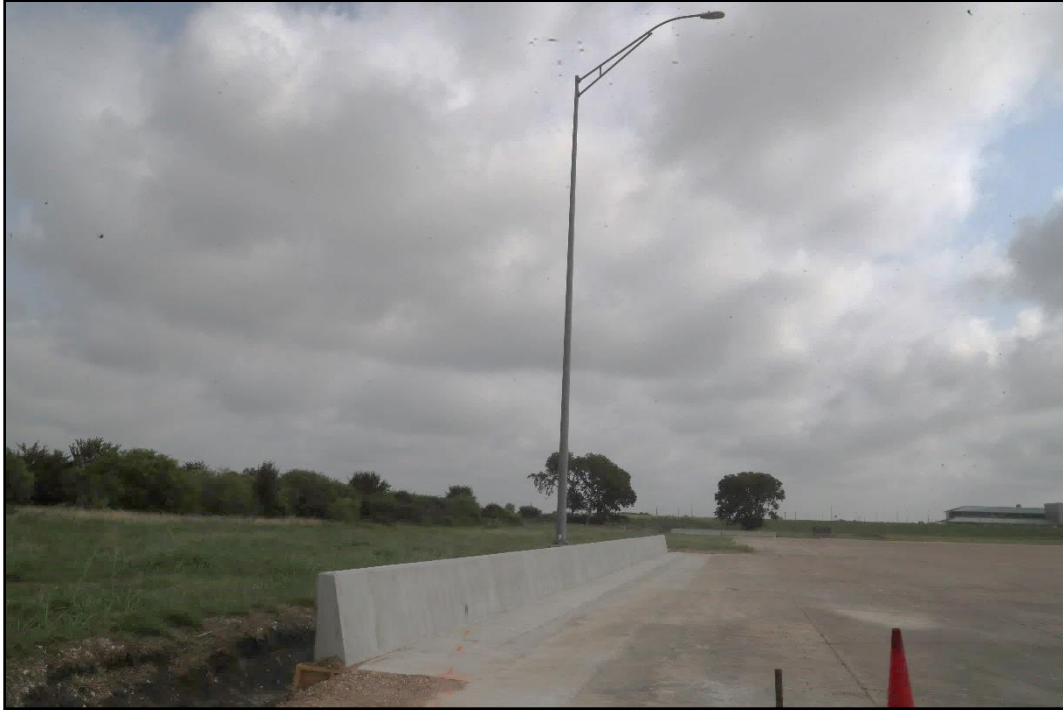
Figure 2.2. Impact Angle on Traffic Side of Luminaire Pole behind Single Slope Traffic Rail Prior to Testing.
