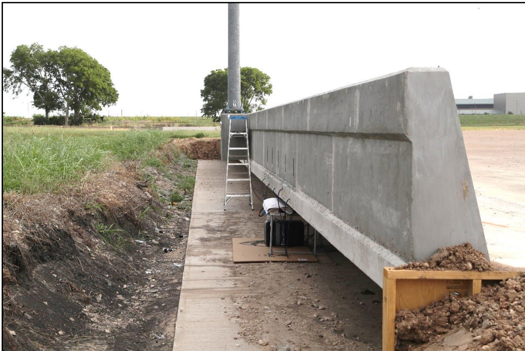
Figure 2.3. Field Side of Luminaire Pole behind Single Slope Traffic Rail Prior to Testing.
