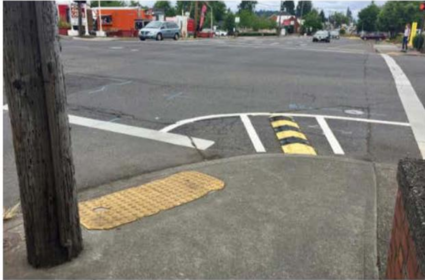
Figure 3.10 Bumps used for right-turn calming in Portland, Oregon (Lindley and Wunderlich, 2023).
