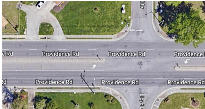
Control Site 2, Intersection A
