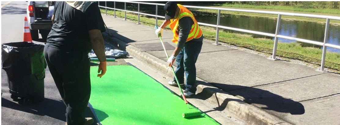
Figure 2-3. Application of MMA Product (NACTO, 2020).
