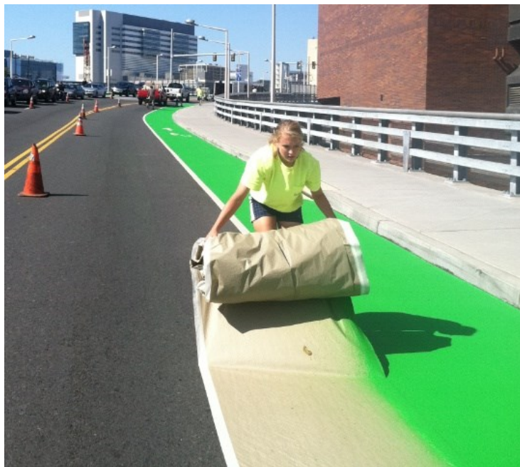
Figure 2-2. New Epoxy Bike Lane Installation, Pennsylvania (NACTO, 2020).
