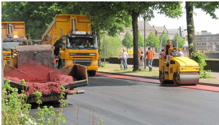
Figure 2-14. Construction of Colored Bike Lane in the Netherlands. (Bicycle Dutch, 2020)
