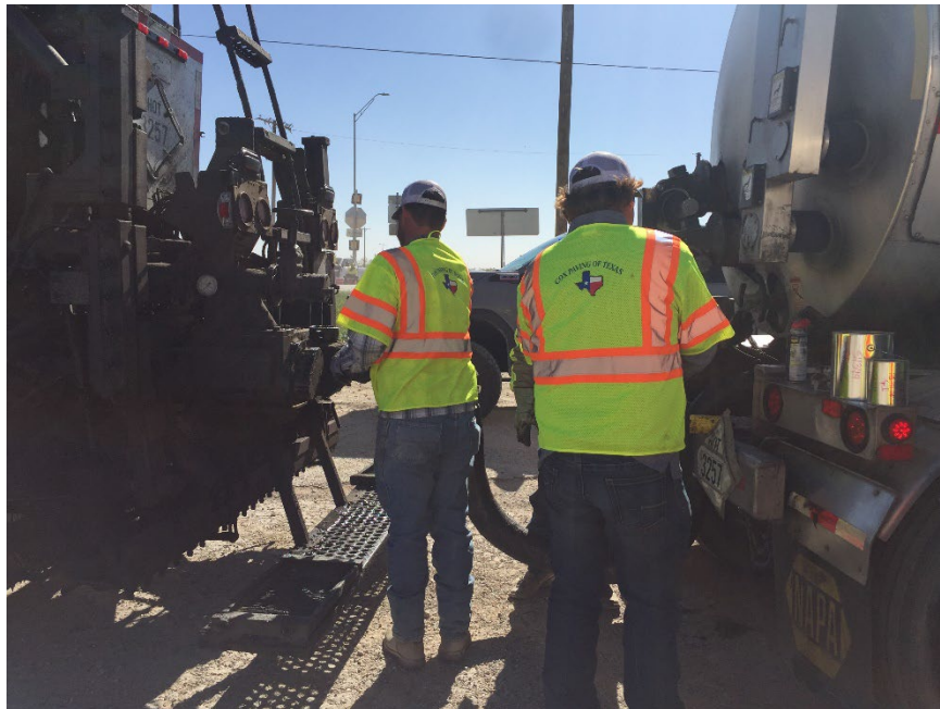
Figure 6. AR Binder Sampling.
