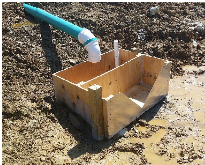
Figure 3-7. Sediment basin outlet 90-degree V-notch weir and box structure used at the Knox and Bedford counties study sites.
