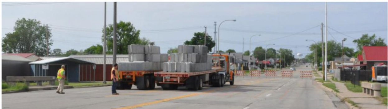
C. Loading bridge at midspan
