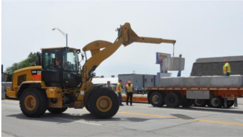
A. Loading trailer with concrete blocks
