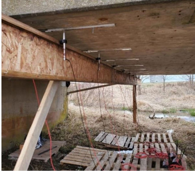
B. Photograph of the fixture with sensors installed on bridge
