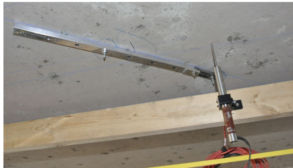
C. LVDT and strain gauge underneath the slab
