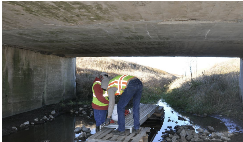
B. Underneath bridge
