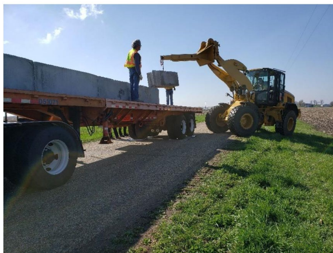
A. Concrete bin blocks used for weight and the crawler crane used to load the trailers
