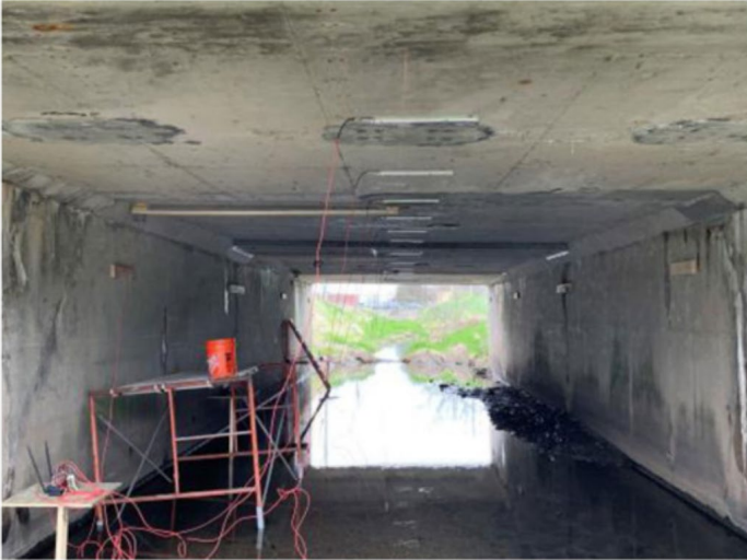
B. Photograph of installed strain gauges
