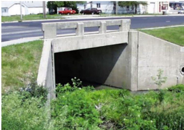
A. Bridge side view
