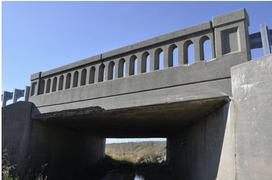
B. Underneath bridge
