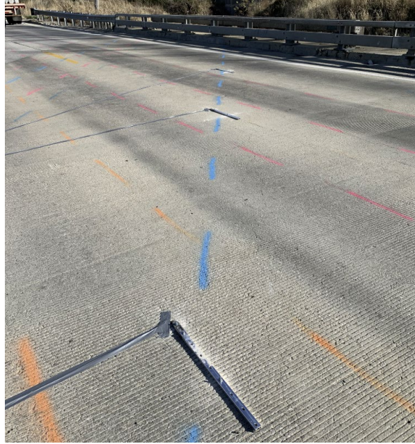
B. Strain gauges above the slab
