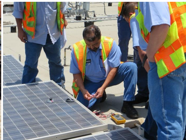
LA Metro staff inspect photovoltaic systems Photo credit LA Metro
