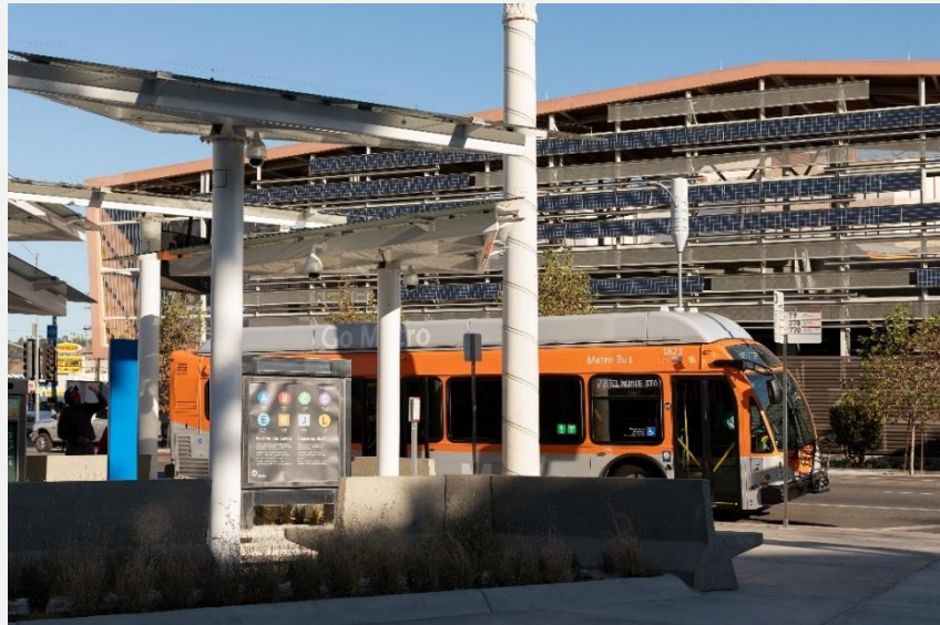
Integration of renewable energy into bus stops. Photo credit: LA Metro
