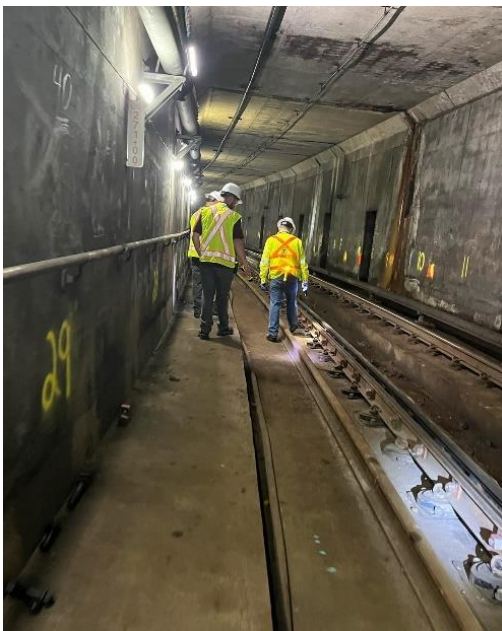
Transit Rail Inspection Photo Credit FTA
