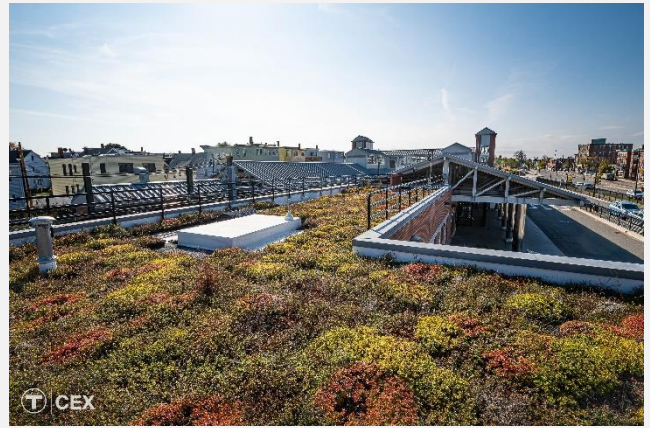
MBTA green roof on Orient Heights Station reduces the amount of stormwater runoff entering the municipal storm system Photo credit MBTA
