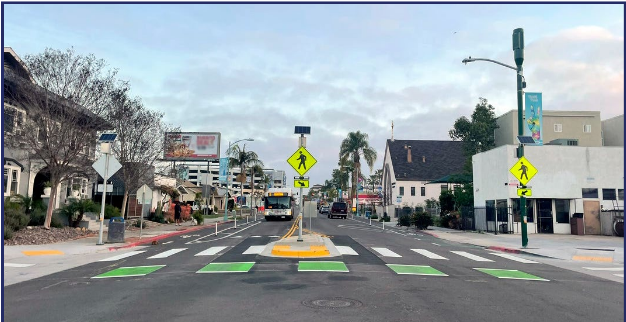
Figure 17. Photo. Example of pedestrian crossing improvements with a rectangular rapidflashing beacons installed at a crossing, along with a pedestrian refuge island.
