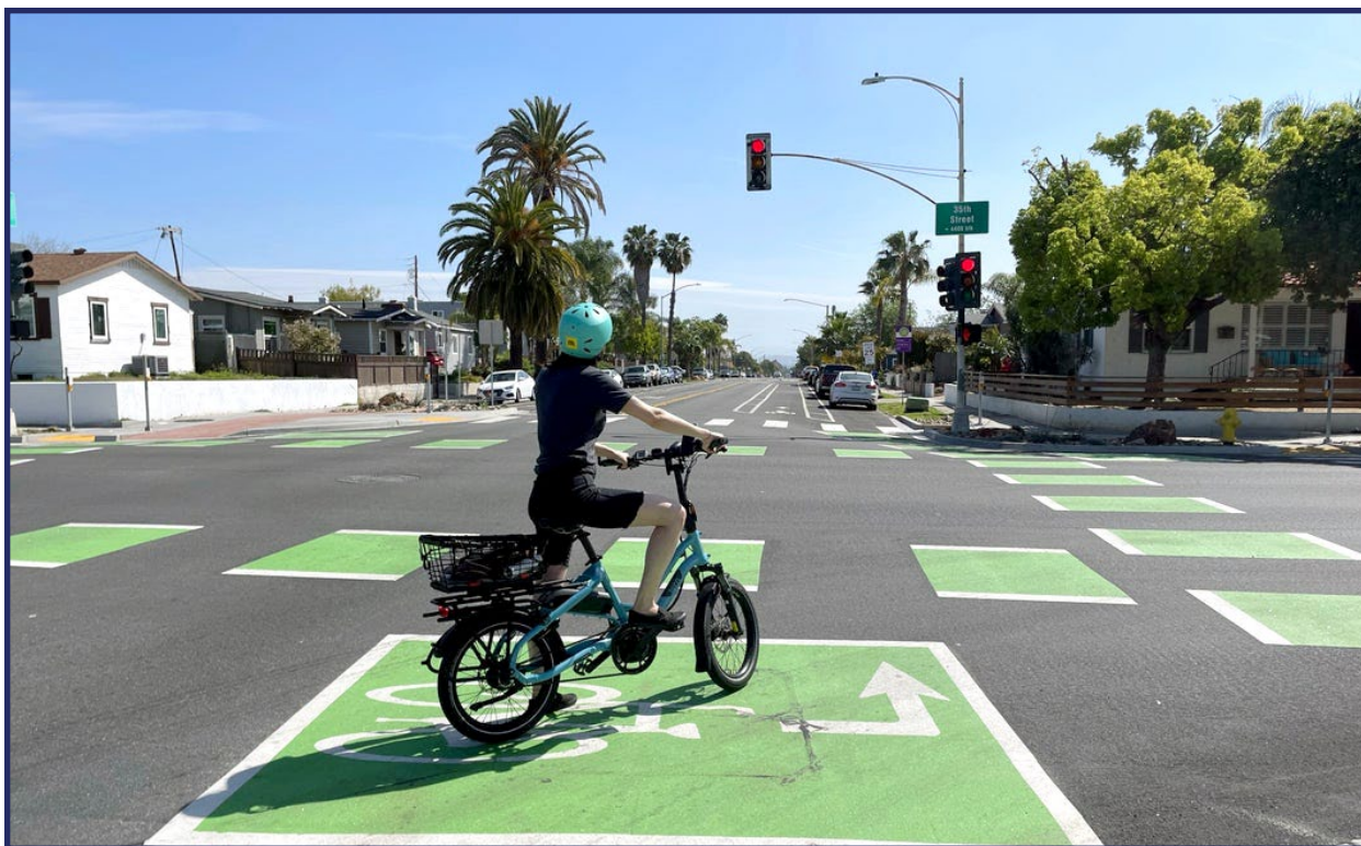
Figure 16. Photo. Example of bicycle-focused intersection improvements in San Diego, CA, with two-stage left-turn boxes providing safe and efficient left-turn opportunities for bicyclists.
