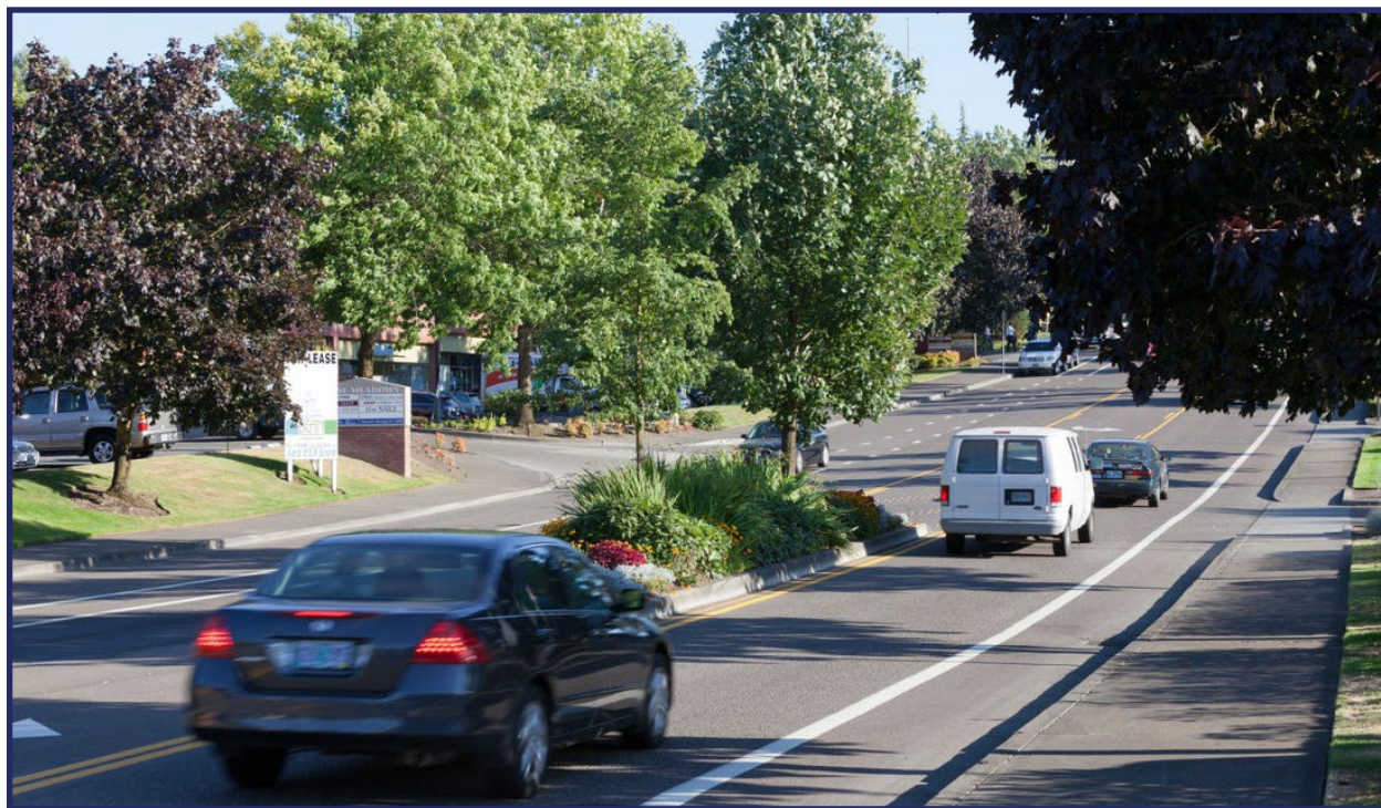
Figure 13. Photo. Example of access management treatments as part of a road diet project that reduces friction and enhances travel and reliability of traffic.
