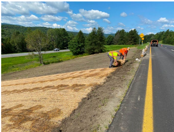
Figures 19: August 22, 2023, Digging a trench to key-in erosion control matting (left); preparing to set erosion control matting (right).
