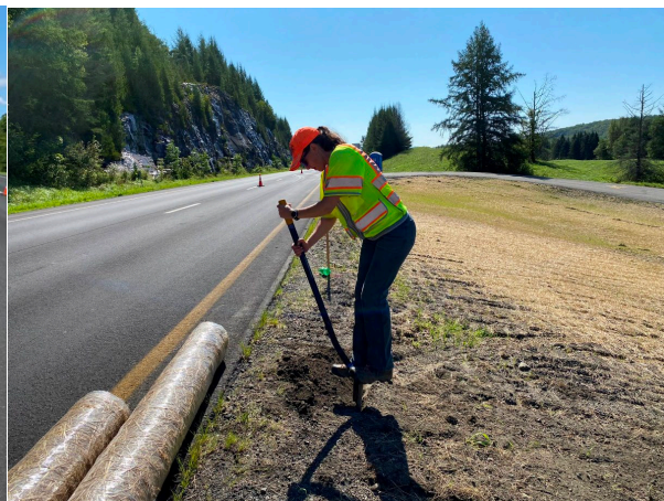
Figures 19: August 22, 2023, Digging a trench to key-in erosion control matting (left); preparing to set erosion control matting (right).
