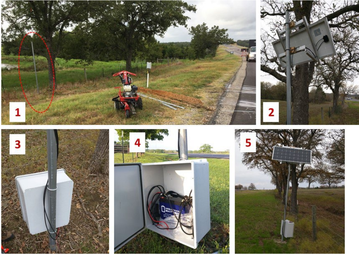
Figure 5.19. Photographs summarizing sequence of installation of power supply components.
