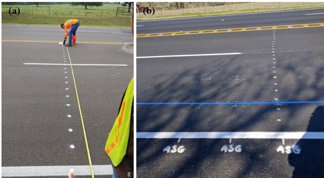
Figure 6.22. (a) Process of marking survey points across the road; and (b) survey points marked on the road (white dots across the road).
