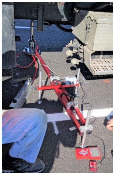
Figure 7.12. UT's static plate load test apparatus with loaded truck as reaction.
