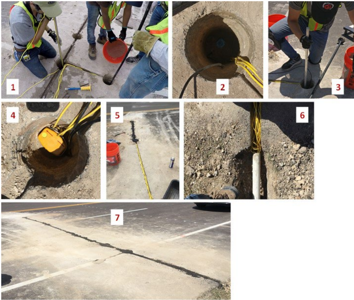
Figure 5.16. Photographs summarizing sequence of geophone installation in base and subbase layers.
