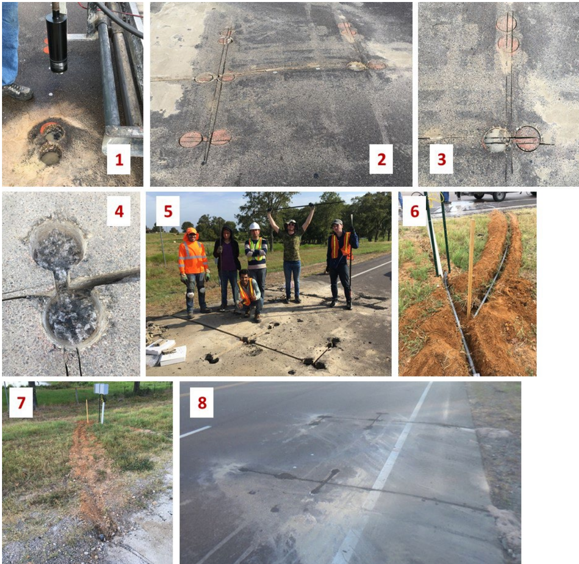
Figure 5.18. Photographs summarizing sequence of ASG installation in preexisting asphalt layer.
