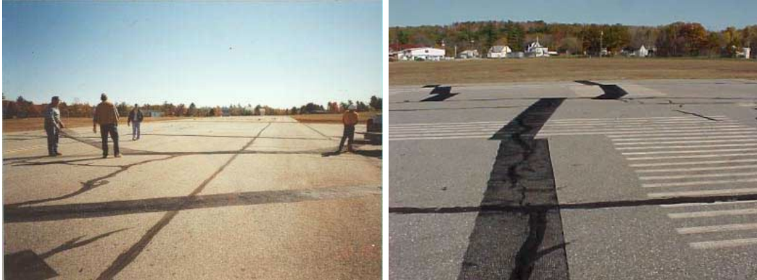
Figure 2.19. Photographs showing the installation of fabrics on transverse cracks (ME 01-3)
