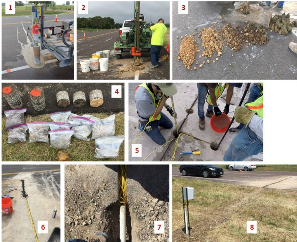
Figure 5.15. Photographs summarizing sequence of moisture sensor installation.
