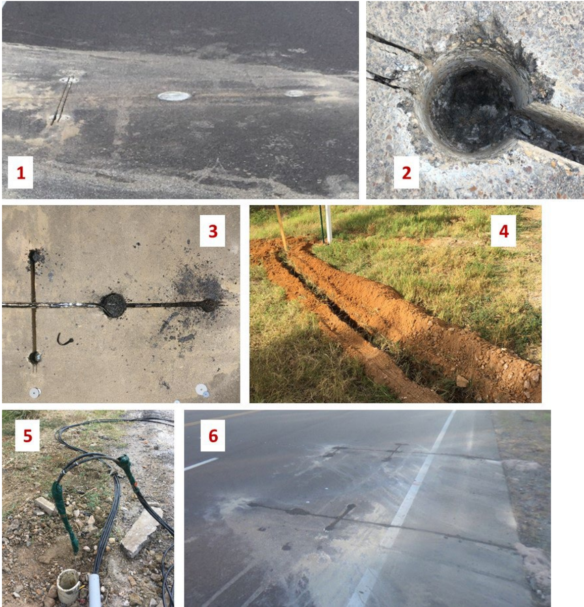
Figure 5.17. Photographs summarizing sequence of geophone installation in asphalt layer.
