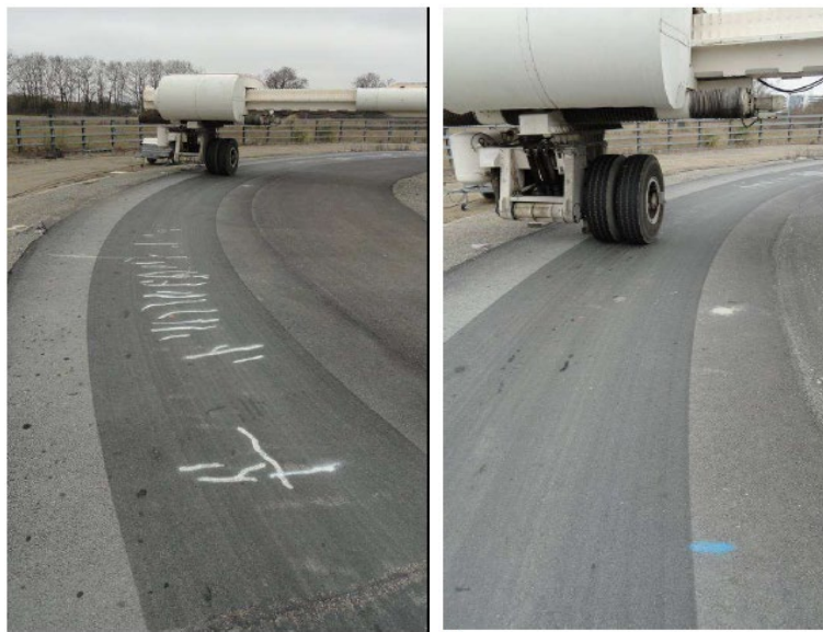
Figure 2.28. Photograph showing control section (left) and fiberglass grid-reinforced section (right) at the end of testing (IFSTTAR, 2012).
