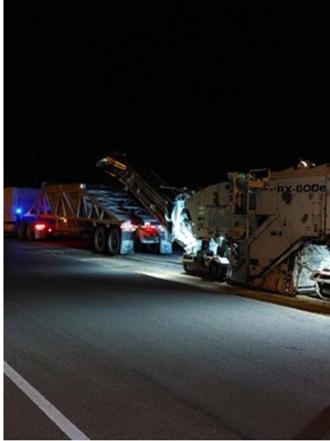
Figure 9.16. Milling of asphalt layer that had fiberglass (FG) geogrid.
