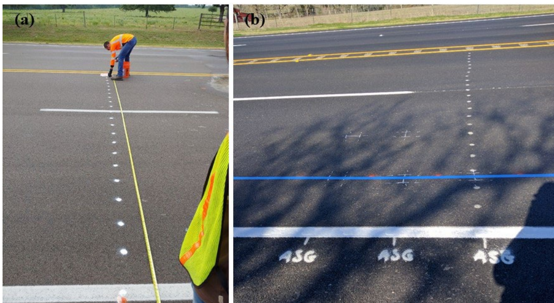
Figure 7.21. (a) Process of marking survey points across road; and (b) survey points marked on road (white dots across road).
