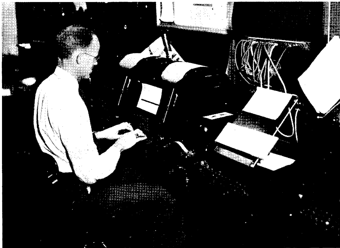
Figure 10.—Interior of a Civil Aeronautics Administration airways teletype station showing teletype-writer machines.
