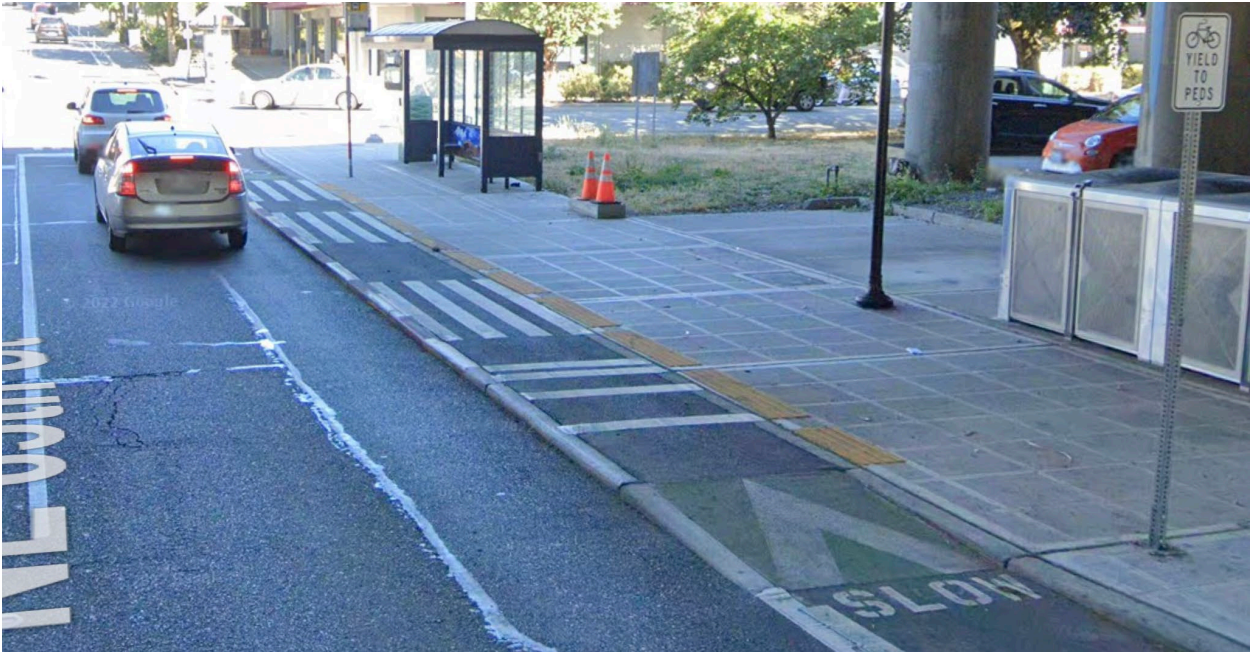
Figure 11 Cycle track bus stop with no additional boarding area. Seattle, NE 65 th Avenue (Source: Google Street View)
