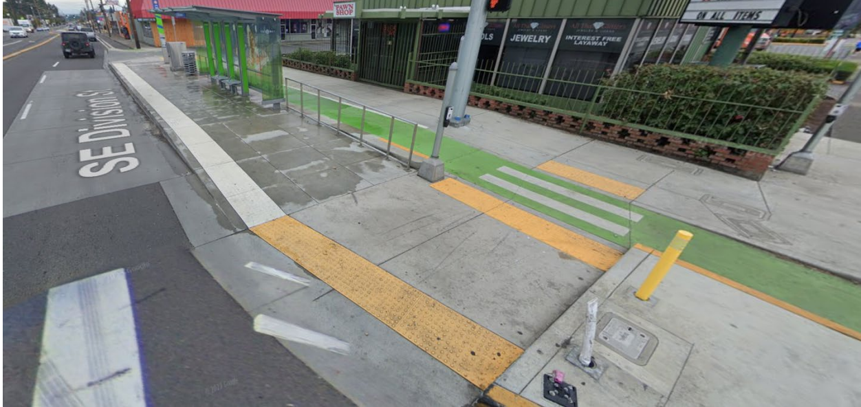
Figure 5 Floating transit island on SE Division and 122 nd Avenue in Portland, OR (Source: Google Street View)
