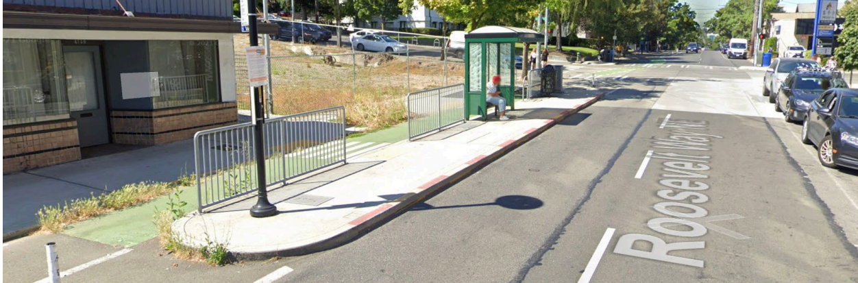
Figure 6 Floating transit island on Roosevelt Way NE in Seattle, WA (Source: Google Street View)
