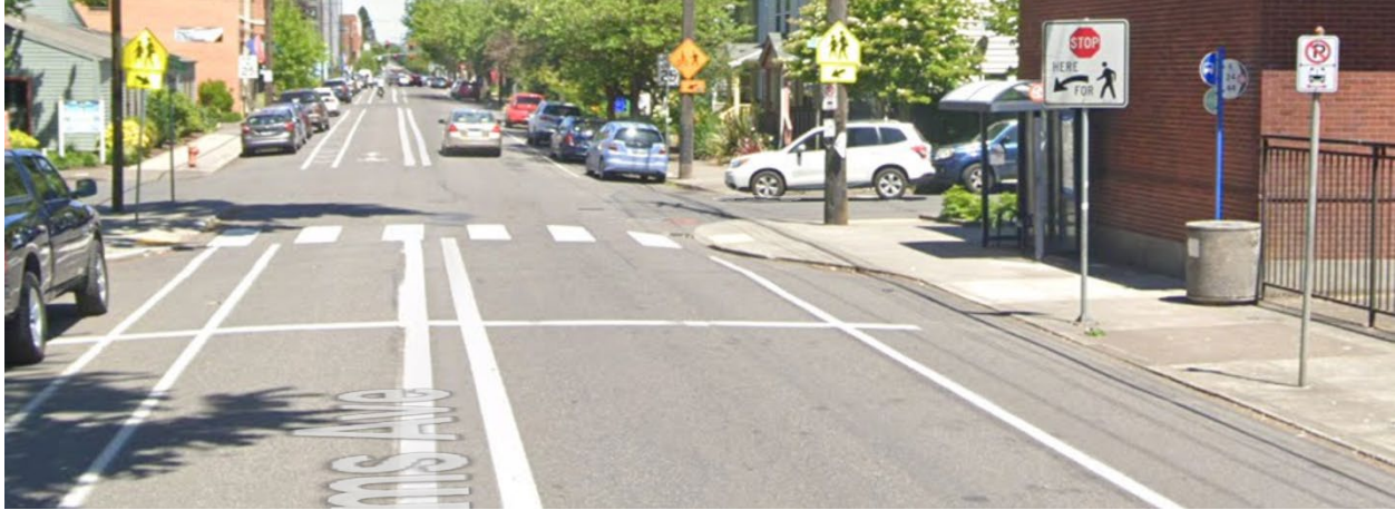
Figure 4 Left-side bike lane with right side bus stop, North Williams Street in Portland, OR (Source: Google Street View)
