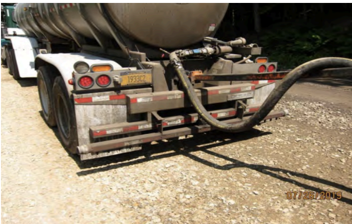
(c) Tanker with calcium chloride and hose to reclaimer
