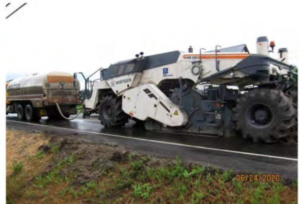
Wirtgen WR250 reclaimer used on the project.
