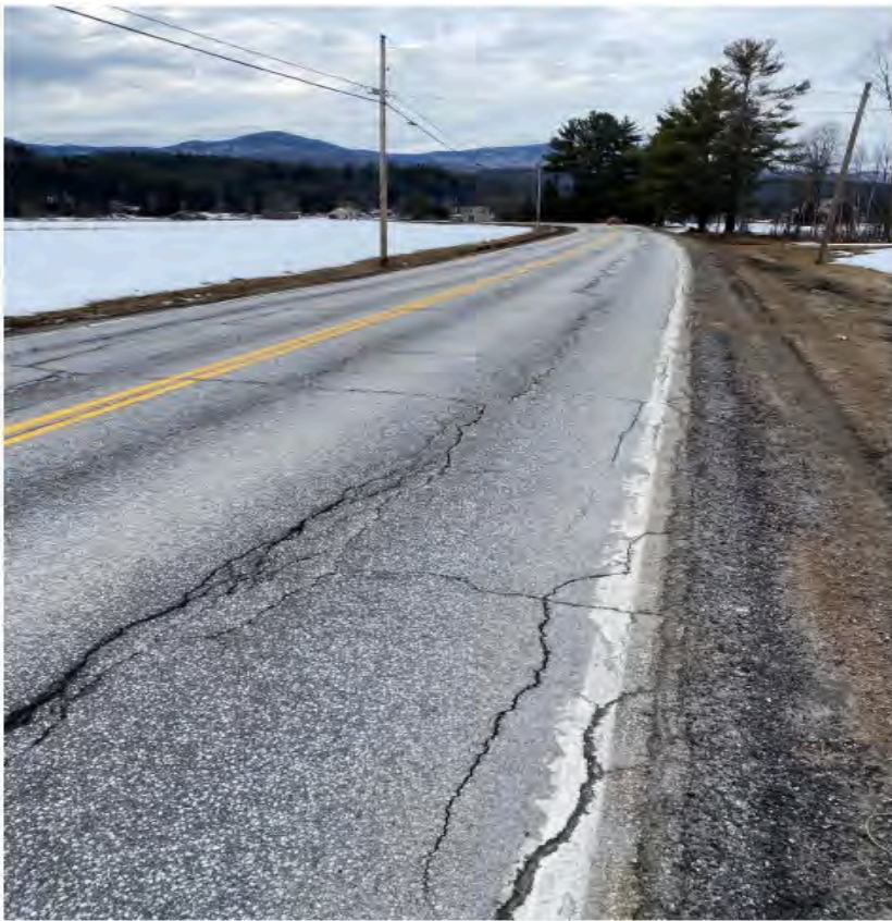
(d) Vermont 12 south of Worcester-Elmore reclaimed stabilized base project March 12, 2020
