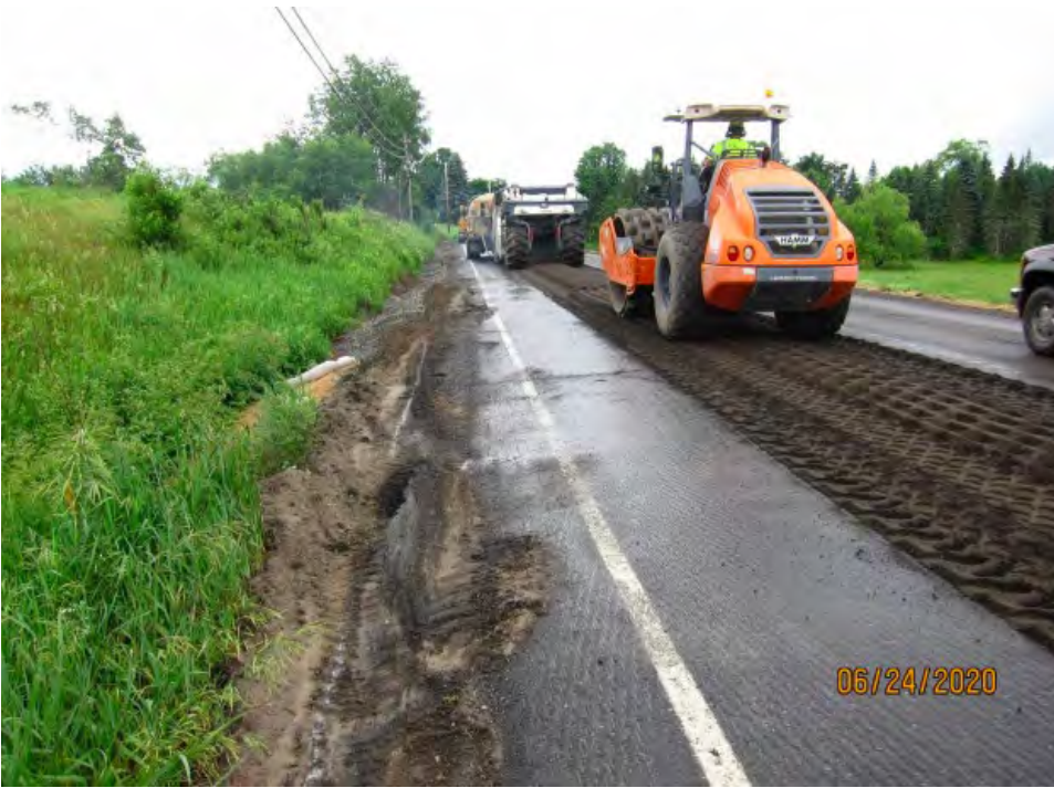
(a) Equipment train with reclaim grinder/mixer supplied by water tanker truck with sheepfoot compactor behind
