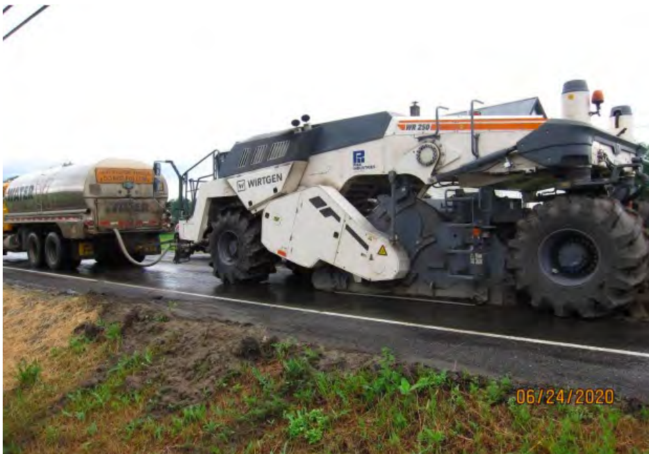
(b) Wirtgen WR250 reclaimer used on the project
