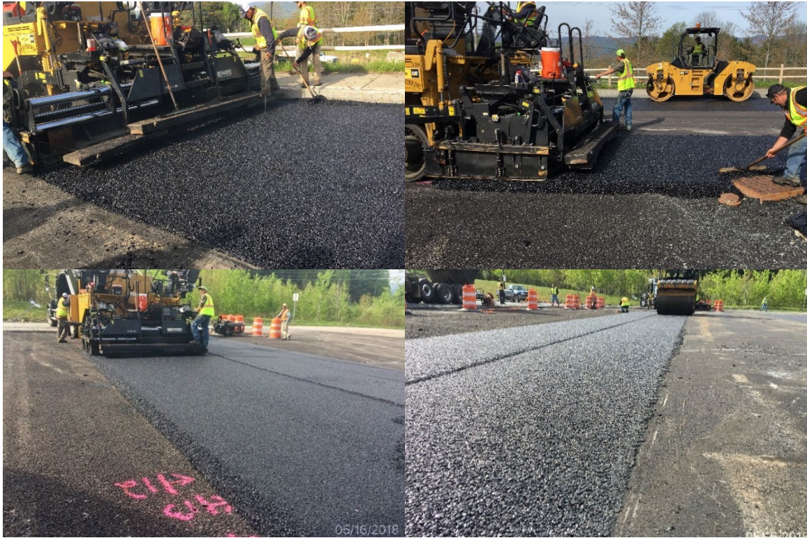
Figure 5: Open Graded Friction Course Paving
