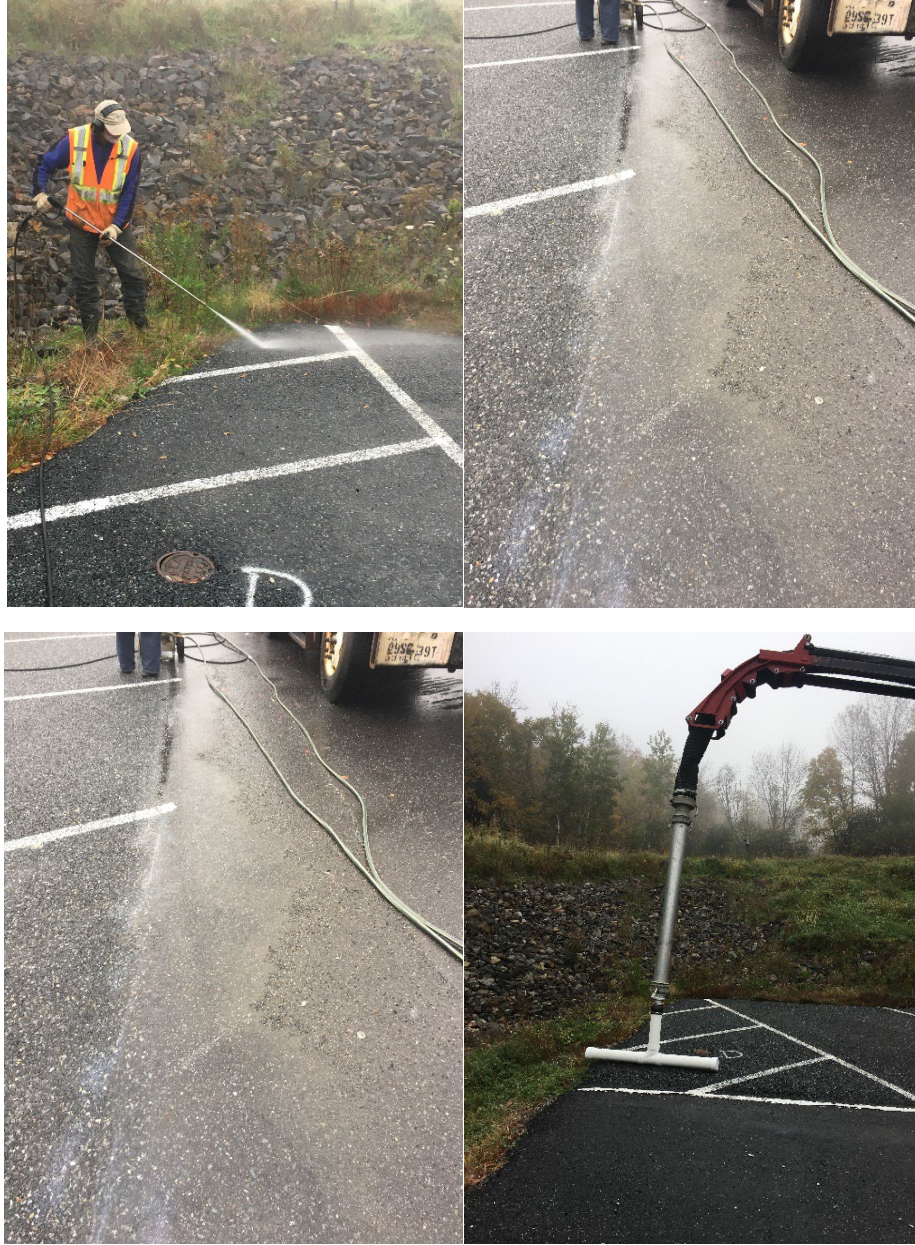
Figure 11: Porous Asphalt Cleaning Procedures
