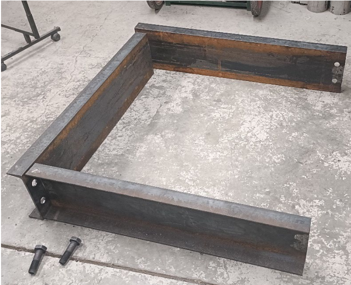
Figure B.1 Preparing the formwork for the upper box
