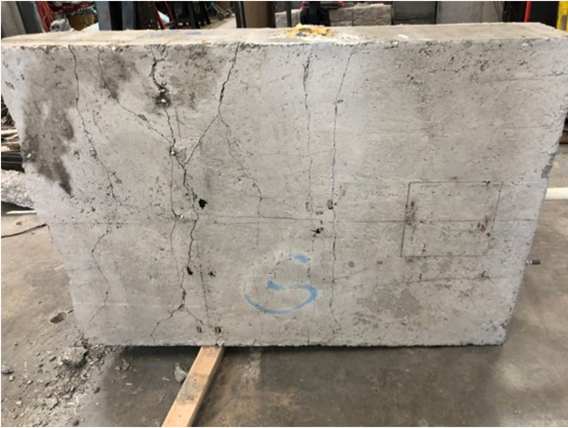
Figure 5.23 Face of GFRP Reinforced Slab After Failure
