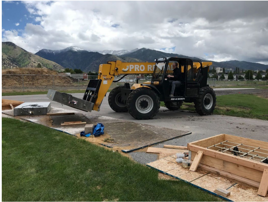
Figure 3.3 Moving the Slabs
