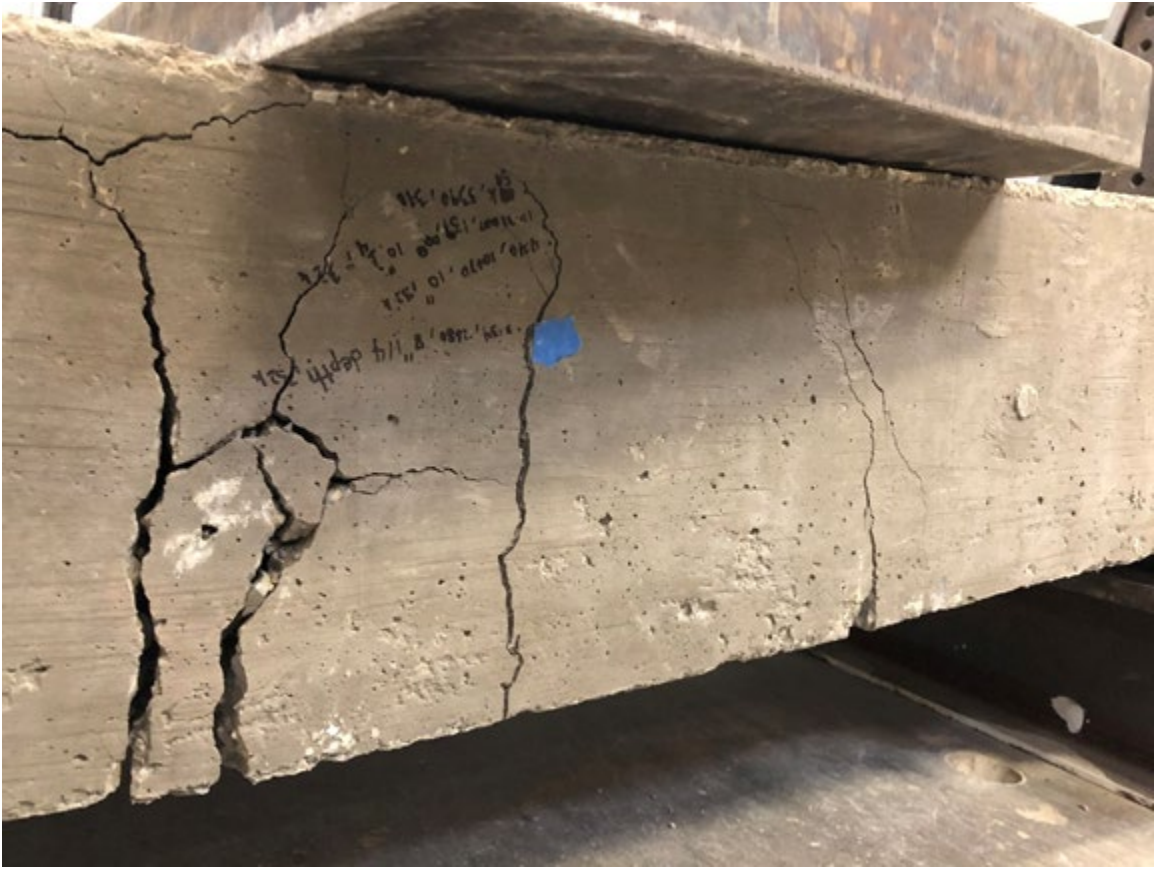
Figure 5.6 Steel Cracks Reverse Side
