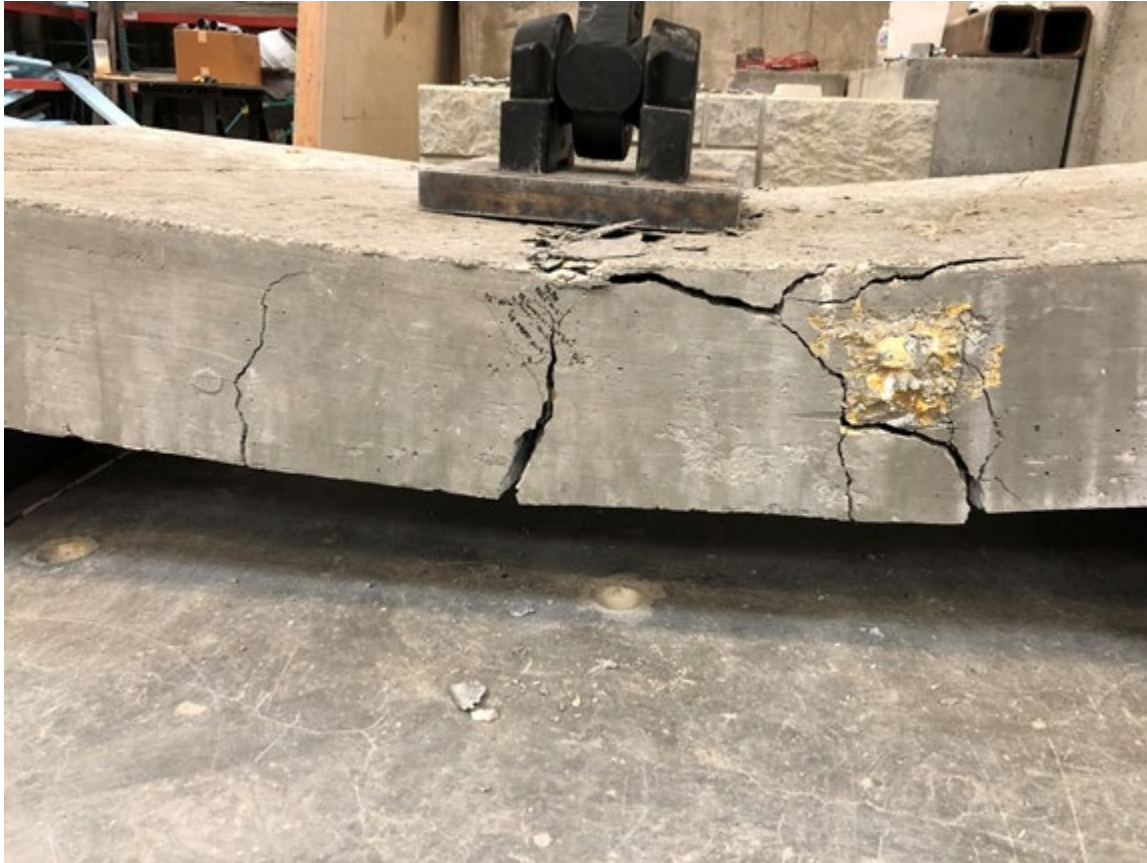
Figure 5.8 Steel Cracking at Midspan
