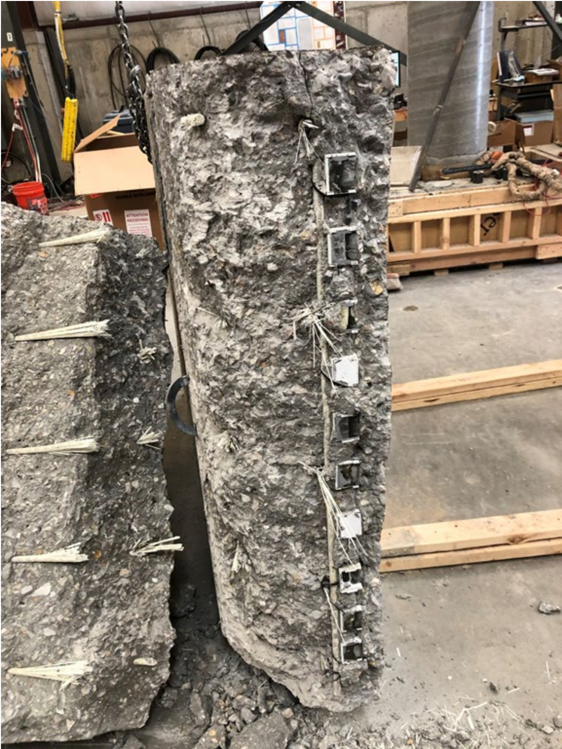
Figure 5.22 GFRP Rupture Exposed
