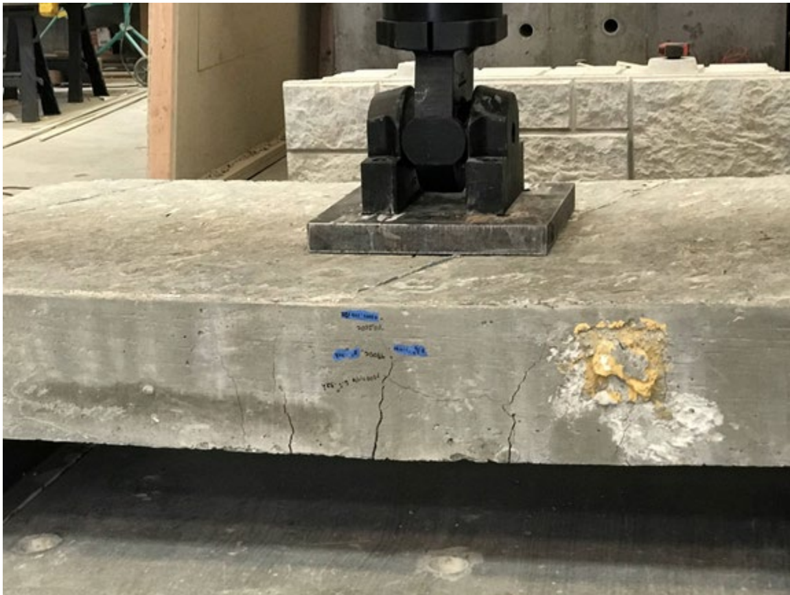
Figure 5.19 Cracking During Static Test
