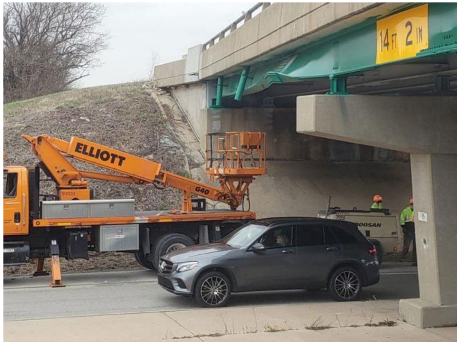
Figure 1. Photo. I-74 bridge over IL-47 on March 26, 2020.
