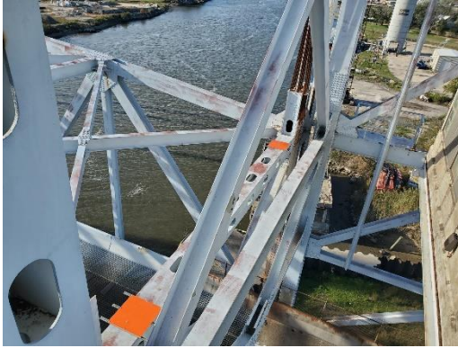
(a) North lift span laser target plates
