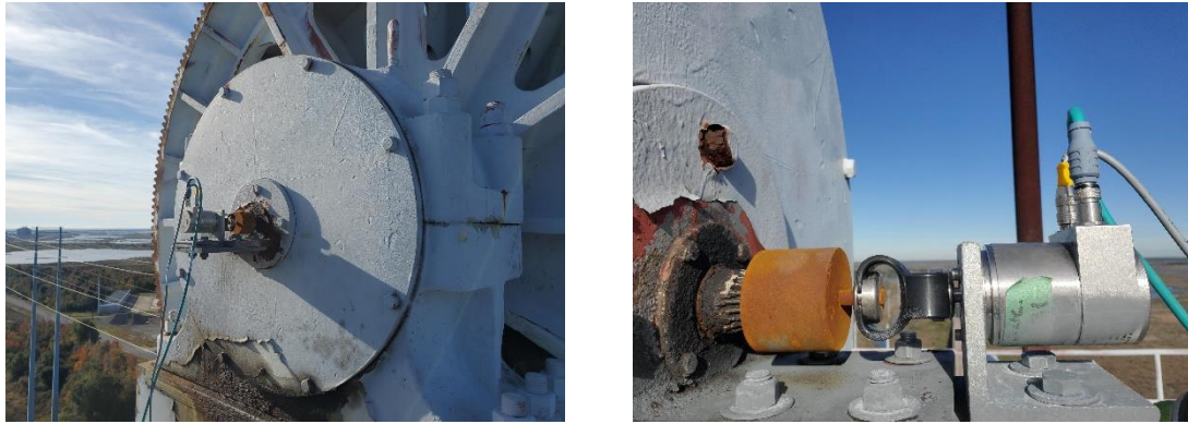
(a) Encoder installation at NW sheave trunnion
