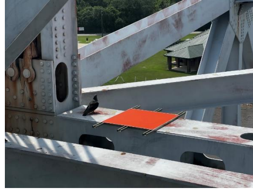
(b) Close up of NE lift span laser target plate
