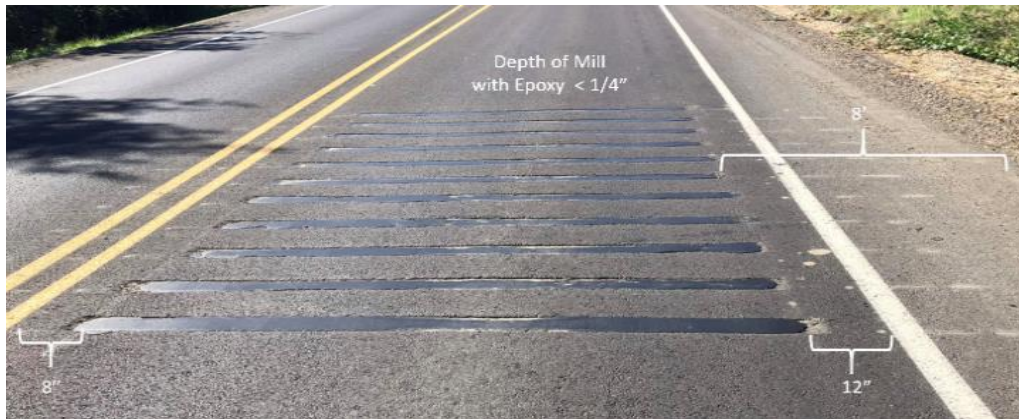
Figure 110. Photo. Epoxy-filled transverse rumble strip.
