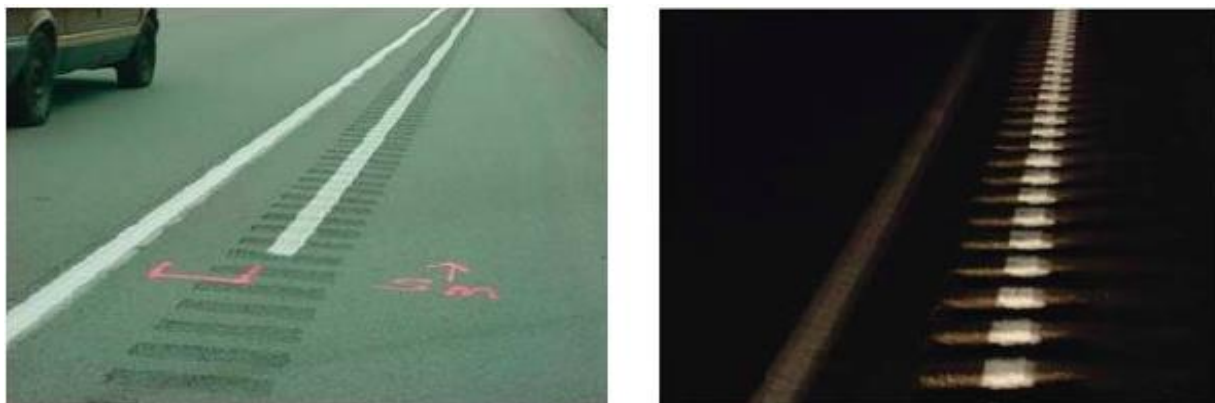
Figure 99. Photo. Daytime and nighttime visibility of edgeline rumble strips.
