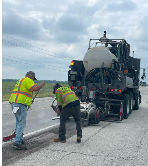
(b) Milling sinusoidal rumble strips
