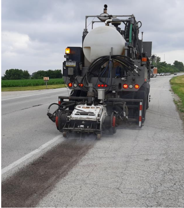
(a) Milling traditional rumble strips
