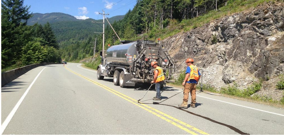
Figure 119. Photo. Crack sealing Application.
