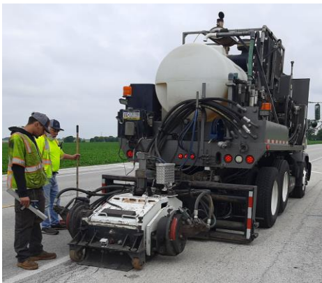
(a) Milling machine for traditional and sinusoidal rumble strips
