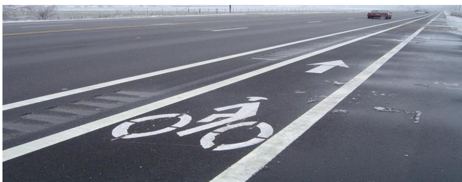
Figure 95. Photo. Rumble strip design with bicycle gap.
