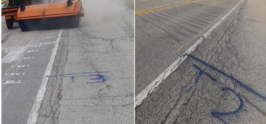
Figure 10. Photo. Marking locations of rumble strips.
