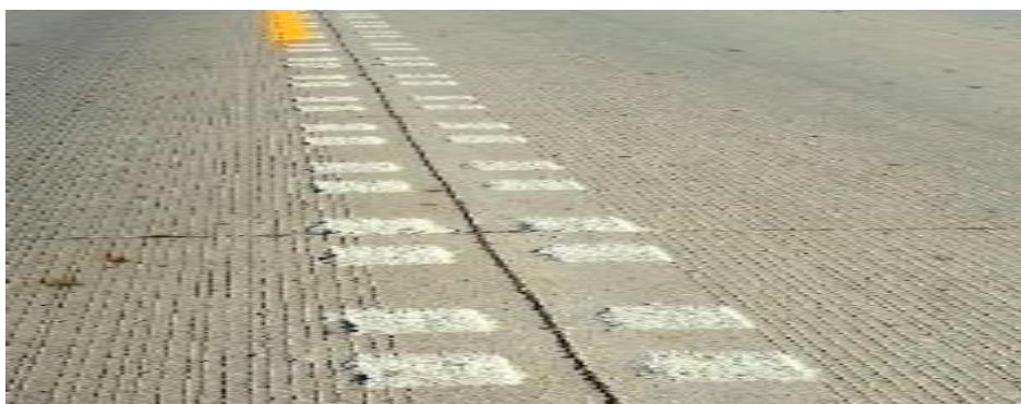
Figure 96. Photo. Rumble strip design with centerline gap.
