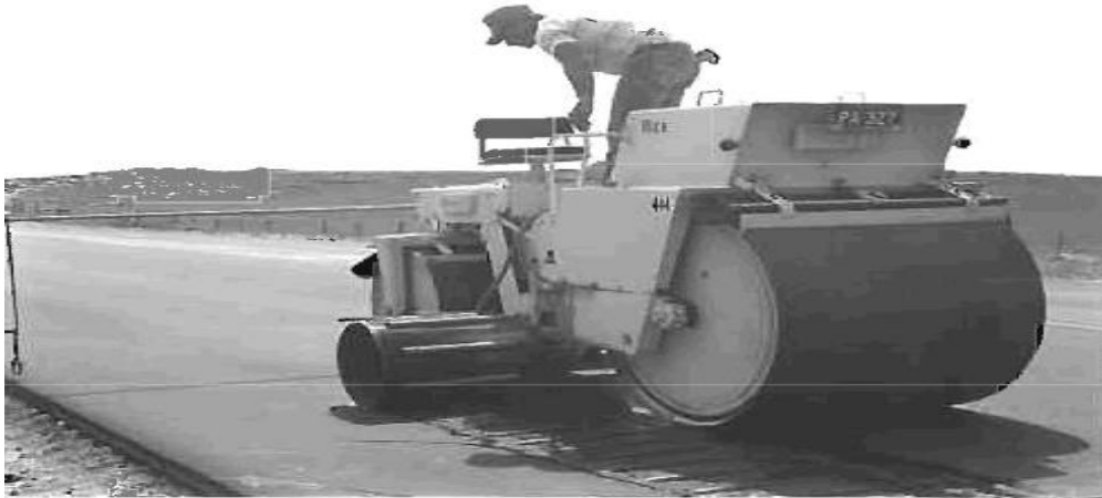
Figure 83. Photo. Rolled rumble strip installation process (Back View).
