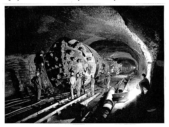
Figure 3-1: Tunnel Boring Machine and Back-up Equipment Assembly
