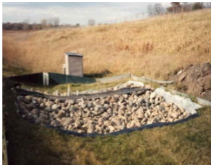
Figure E.5 Pollution control research showing the check dam at MnROAD (4)
