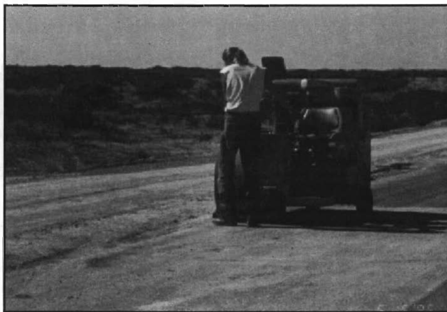
Figure 4.3 Shotblasting equipment
