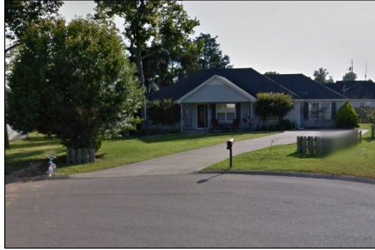
Figure 2. Driveway of incident site. May 2013 image obtained from an internet-based mapping system.
