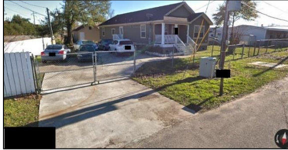
Figure 3. Street view of the incident site viewed in a southwesterly direction. January 2019 image obtained from an internet mapping software.
