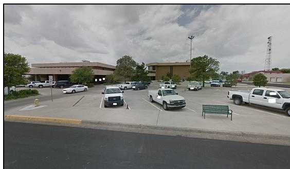
Figure 1. Incident site, looking west (Google Maps image)
