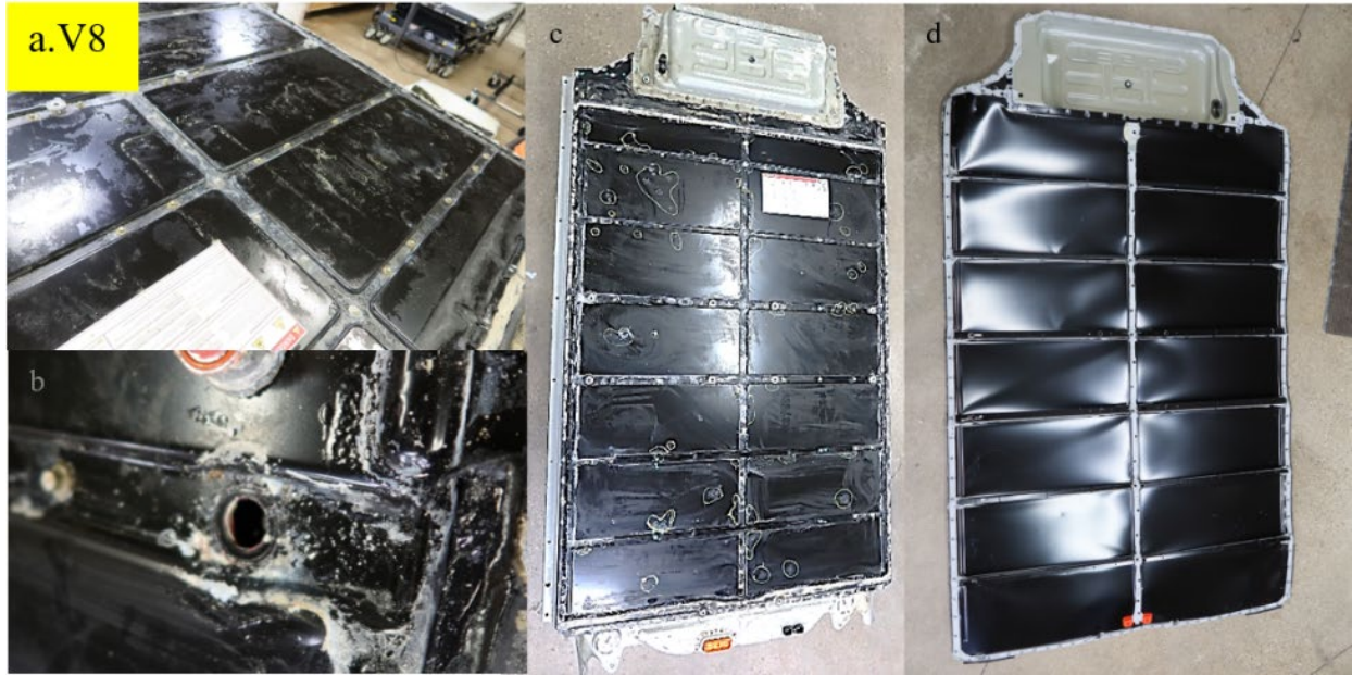
Figure 37. V8 battery pack after removal from the vehicle: (a) water underneath plastic cover, (b) salt residue near a fastener, (c) marked corroded areas, and (d) corrosion free lid underside
