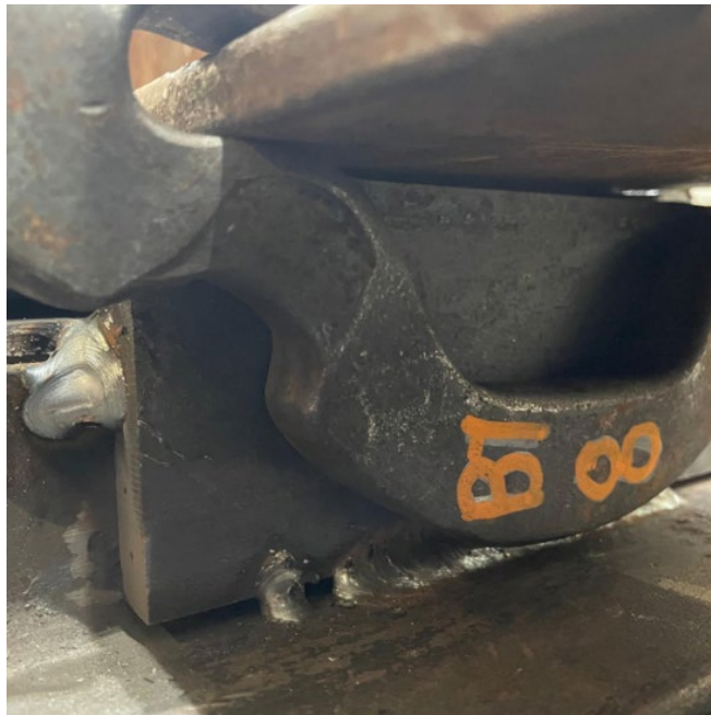
Figure 3: Rail, tie, and anchor
