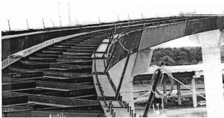
Figure 1. 4 Erected u-shaped girders prior to deck placement
