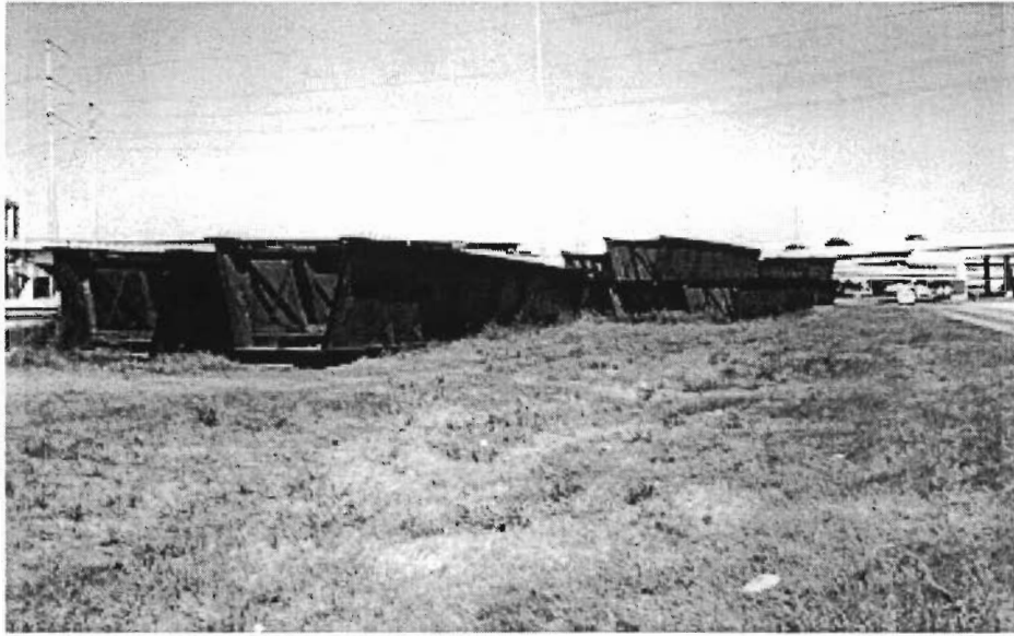
Figure 1.2 U-shaped girders prior to erection
