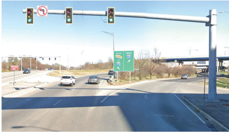
Figure 4.1 Picture of the West St. ramp.
