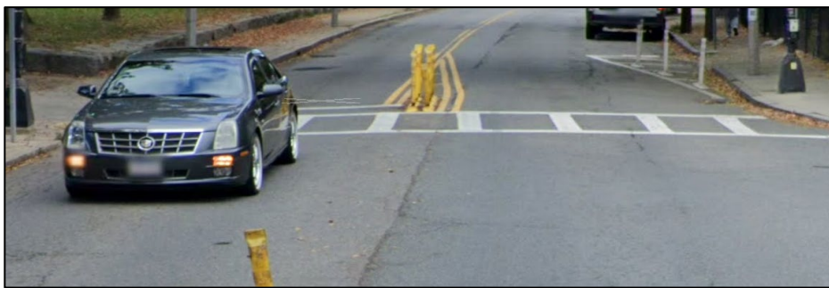
Figure 2.18: Centerline or corner hardening, Boston, MA
