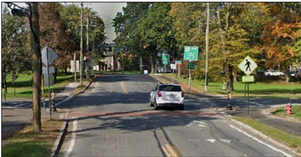
Figure 2.10: Mainline crossing table, Amherst, MA
