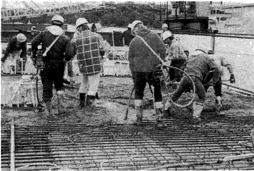
Figure 1.3 Consolidation of concrete in bridge deck
