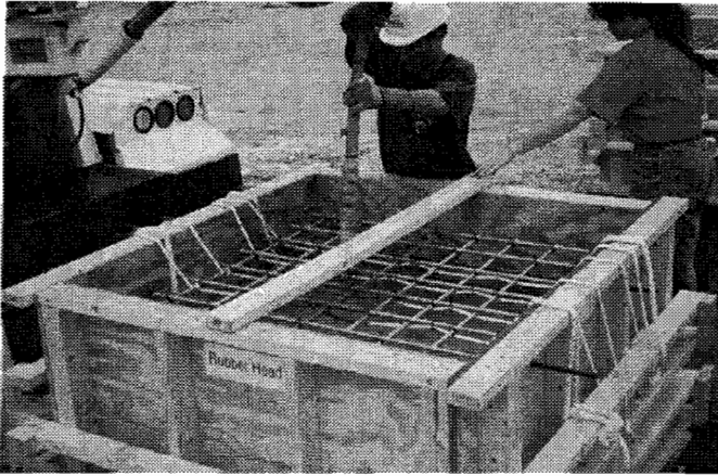
Figure 2. 12 Consolidating footing specimen
