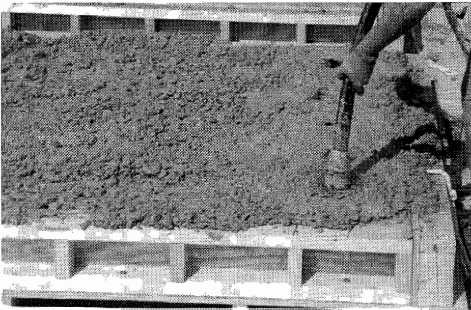
Figure 2. 15 Consolidating slab specimen
