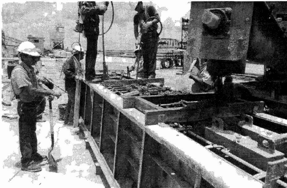
(b) Vibration of concrete in precast element
