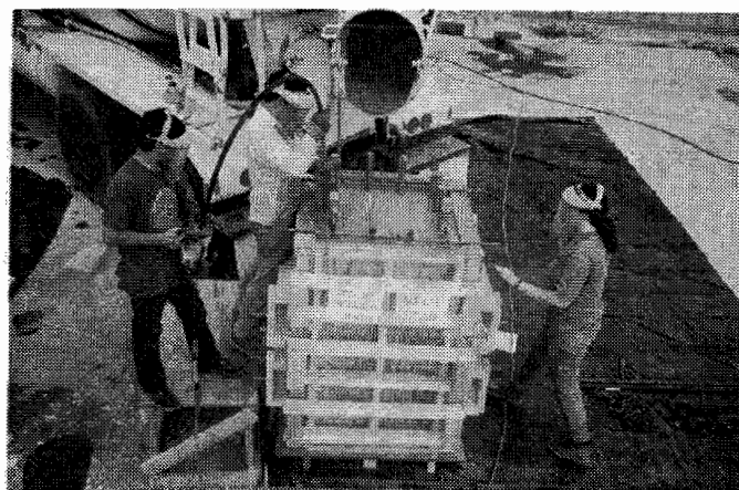
Figure 2.8 Consolidating column specimen
