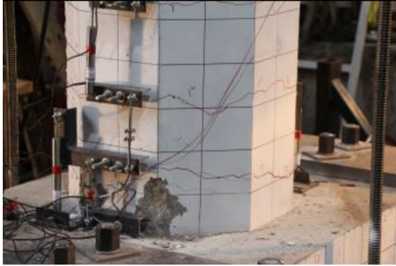
(a) Drift ratio=3% (cracks and spalling)
