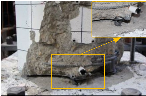
(c) At the end of test (spalling, exposed rebar cage, and fractured bar)
