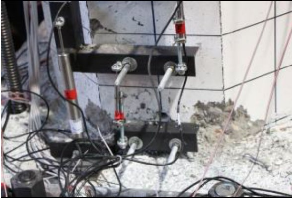
(a) Drift ratio=3% (cracks and spalling)
