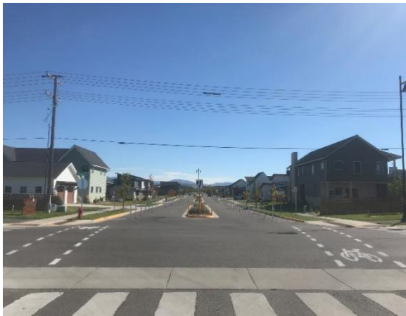
Appendix A Figure 9 Pop-up bike lanes on Annie St in Bozeman, MT
