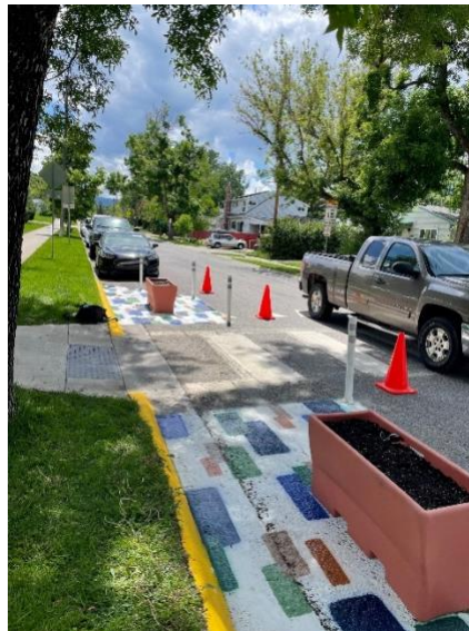
Appendix A Figure 10 Curb extensions with street art on Church St in Bozeman, MT
