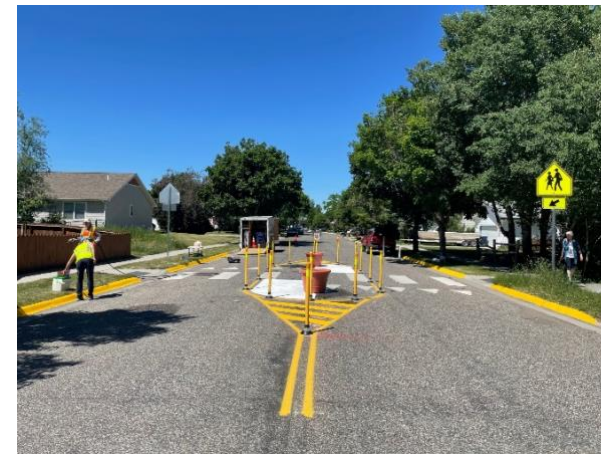
Appendix A Figure 11 A pedestrian refuge island on Ravalli St in Bozeman, MT
