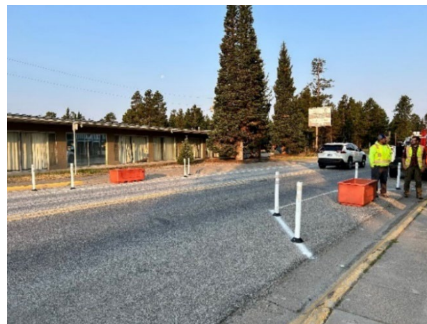
Figure 2 Hwy 20 Curb Extension with W. Yellowstone Staff
