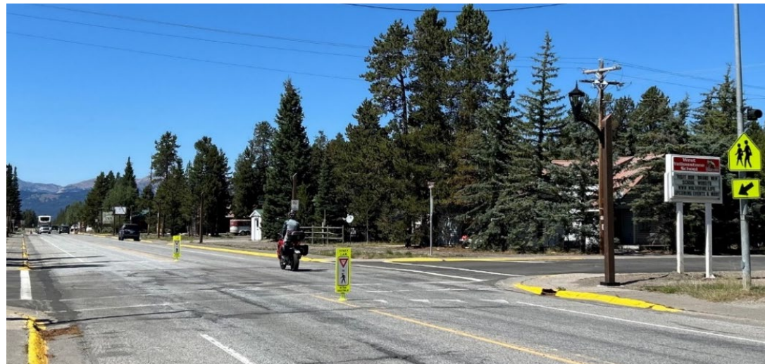
Figure 4 In Road Yield Signs (R1-6) at Hwy 20 & Geysir Intersection
