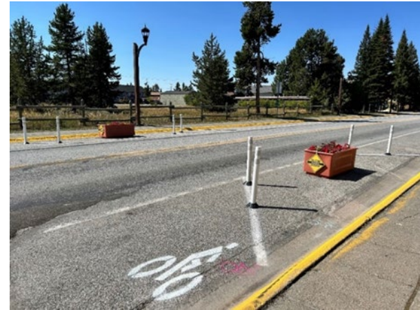
Figure 3 Adjusted Curb Extension with Bike Lane
