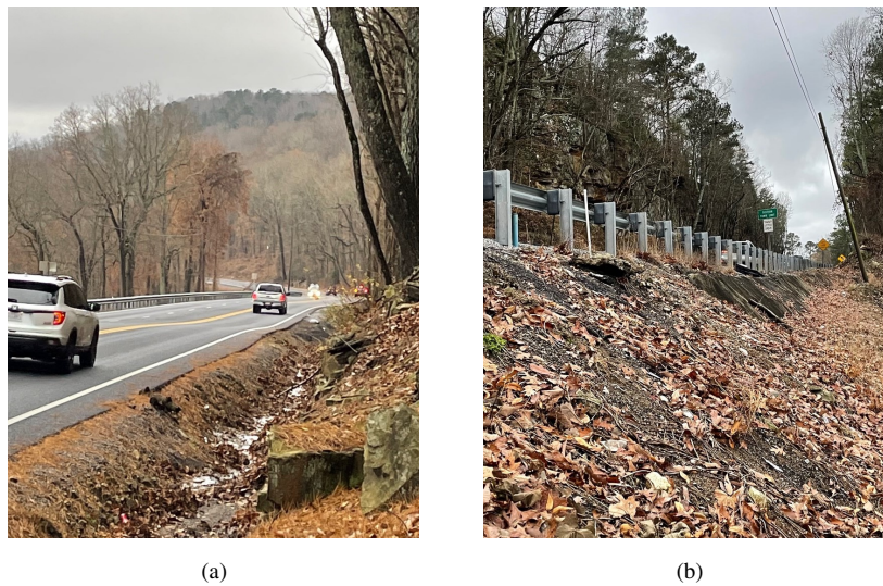
Figure 10: Photos from the monitored site on SR-35 in Jackson County, north of Section, AL. Figure a (facing northeast) shows a vertical offset in the roadway, where the scarp of the slide likely crosses the highway, and the drainage ditch on the south side of the road. Figure b shows the location of original instrumentation along the southbound guardrail.
