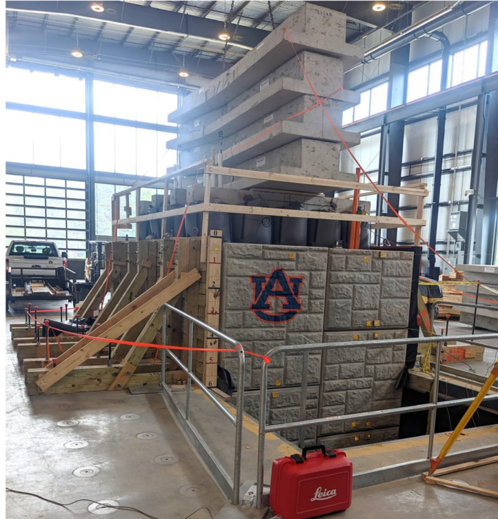
Figure 18: Photo showing the MSE wall at the end of load testing with all imposed surcharge loads (Okafor 2024).
