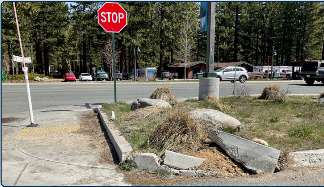
Figure 12: Streetscaping damaged by winter plows (Image Source: City of South Lake Tahoe).
