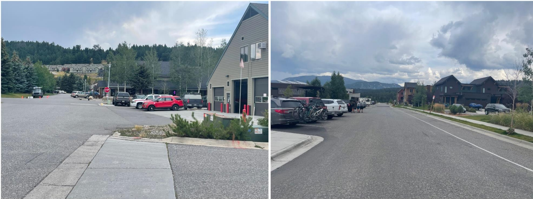
Figure A-4: Where the sidewalk ends on Aspen Leaf west of Ousel Falls Road (left). Aspen Leaf Road looking east towards BASE.
