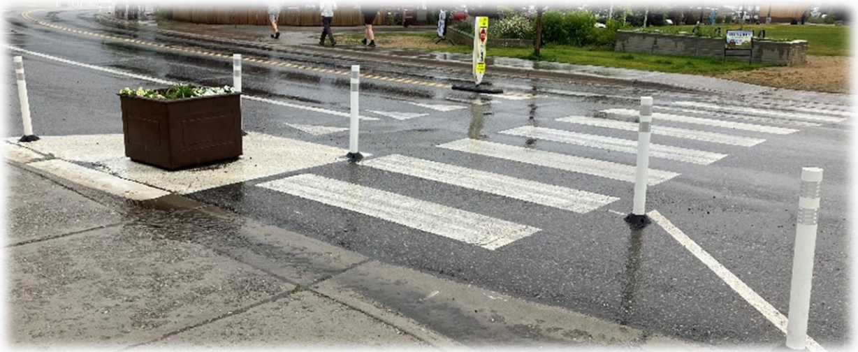
Figure 16. Transit stop curb extension on Ousel Falls Rd.
