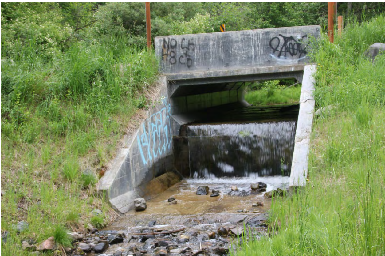
Figure 45 Aquatic Passage Assessment: The picture shows a culvert designed as a fish barrier
