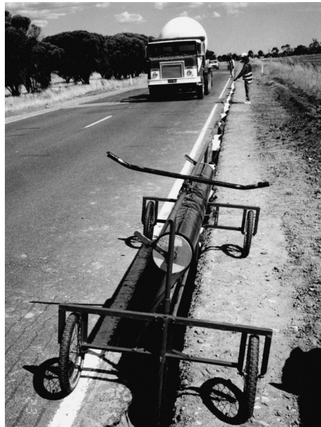
Figure 30: Installation of a Vertical Moisture Barrier (Evans and McManus 1999)
