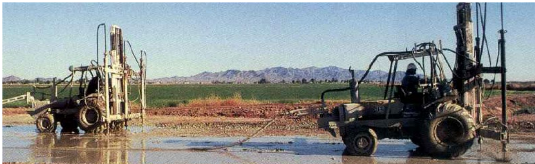
Figure 39: Rubber Tired Injection Machines Used in the Belloat Road Project (Hayward Baker 1990)
