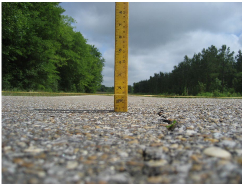
Figure 62: Observed Rutting Near Boring 5.0 MP 52.85 (Rut Depth 1\frac{3}{8} inch) (Photo Taken 09/13/16)
