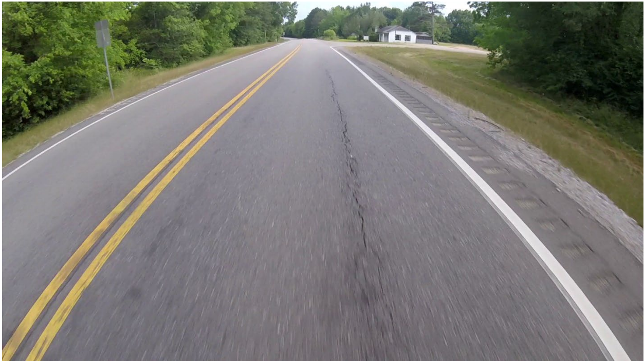
Figure 216: Cracking in Control Near Tree
