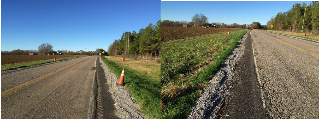
Figure 135: Installed Edge Drains
