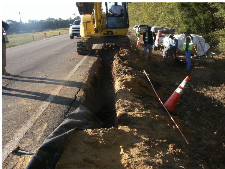
Figure 120: Vertical Moisture Barrier Filling
