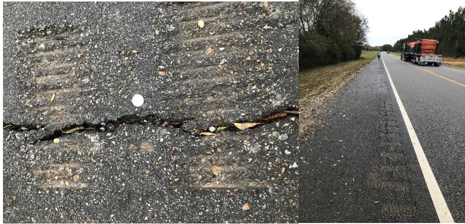
Figure 203: Cracking in the paved shoulders section
