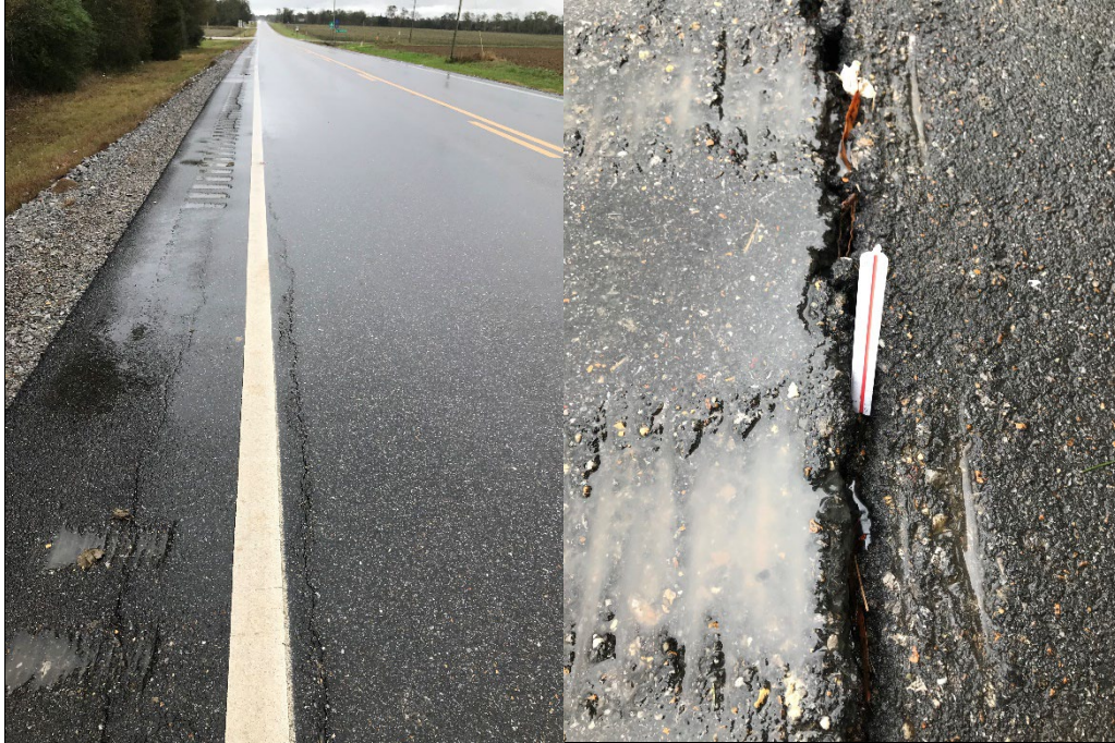
Figure 205: Vertical barrier section crack propagation
