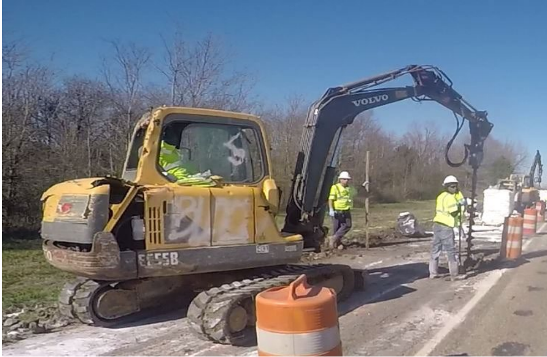
Figure 124: Lime Column Drilling
