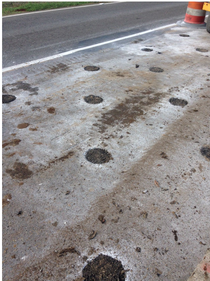
Figure 127: Cold Mix Patching Completed Lime Columns
