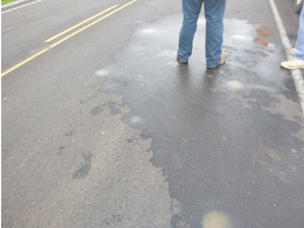
Figure 128: Lime Columns Reflecting to Pavement Surface
