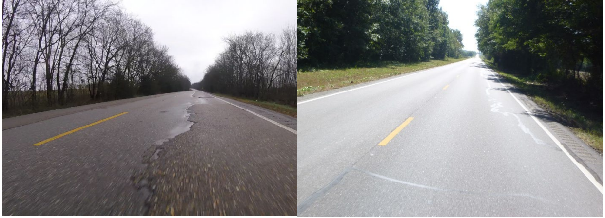
Figure 200: Tree related distress on AL in Dallas County
