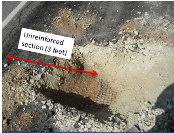
Figure 41: Picture of Excavation and Geogrid Edge (Zornberg and Gupta 2009)
