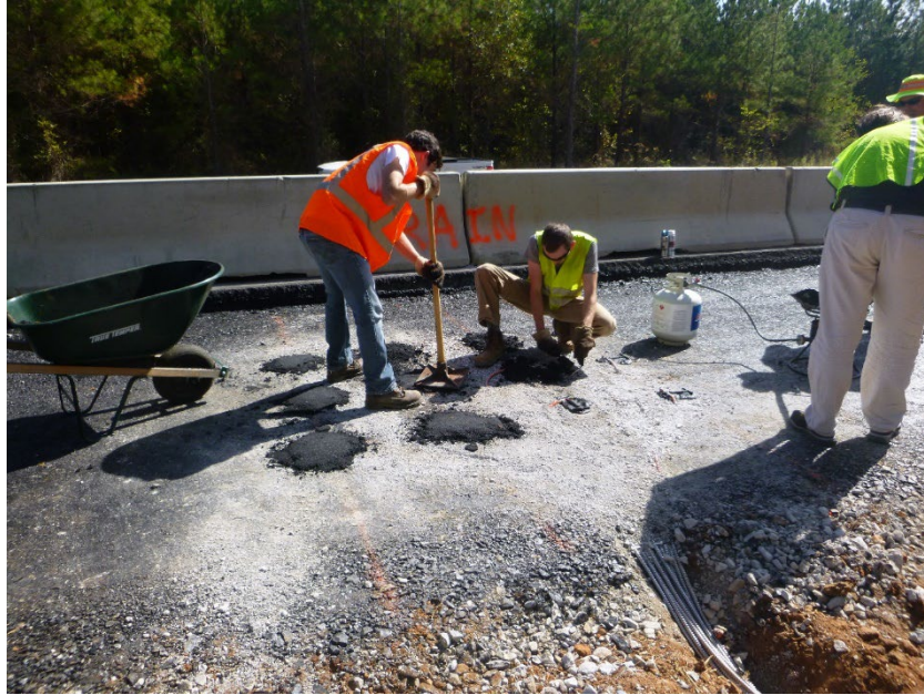
Figure 164: Screened Asphalt being Placed and Compacted over Gages
