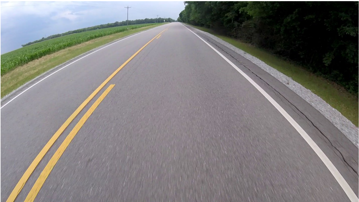
Figure 220: Opening Crack with Settlement in Safety Widening of Paved Shoulders
