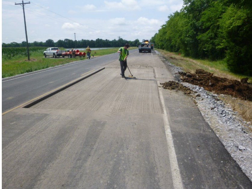
Figure 165: Section Milled and Cleaned for placement of ASG Array
