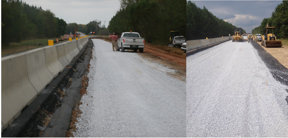
Figure 112: Sand Blanket Drainage Plane Material
