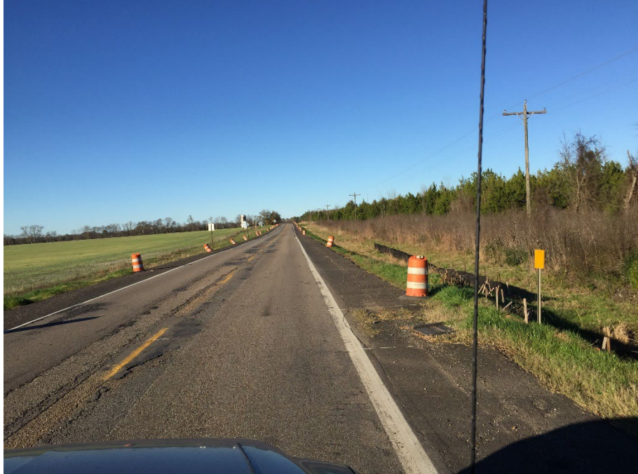
Figure 131: Longitudinal Cracks in Travel Lane at AL 5 Visible During Construction
