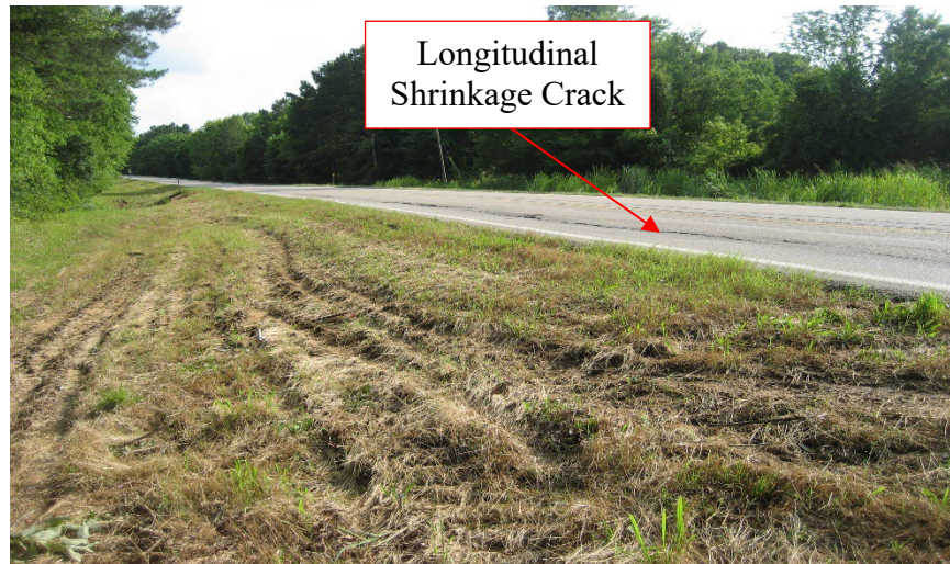
Figure 59: Longitudinal Crack due to Shrink Swell near Boring 5.0 MP 52.85 (Photo Taken 06/02/15)
