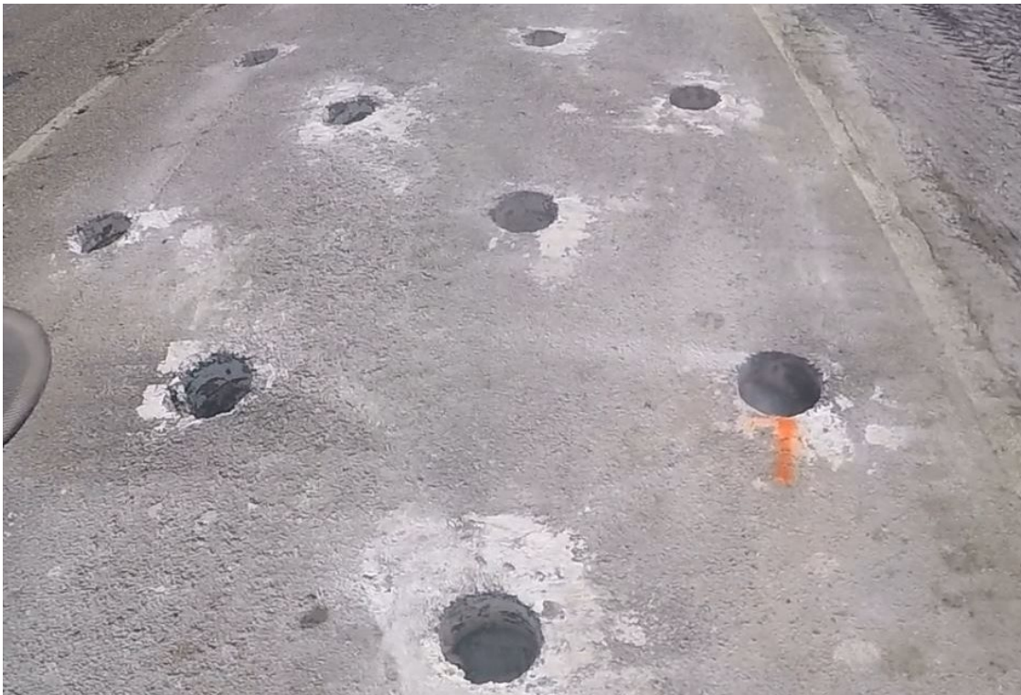
Figure 125: Lime Column Drilled Holes
