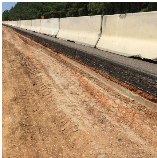
Figure 111: Excavation for Sand Blanket Showing Thick Pavement Over Minimal Compacted Base
