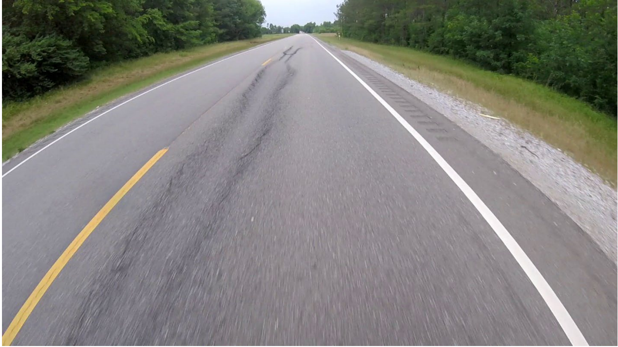
Figure 221: Pavement Surface Raveling in Control Section
