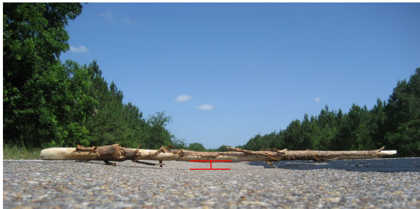
Figure 64: Observed Rutting (Photo Taken 09/14/16)
