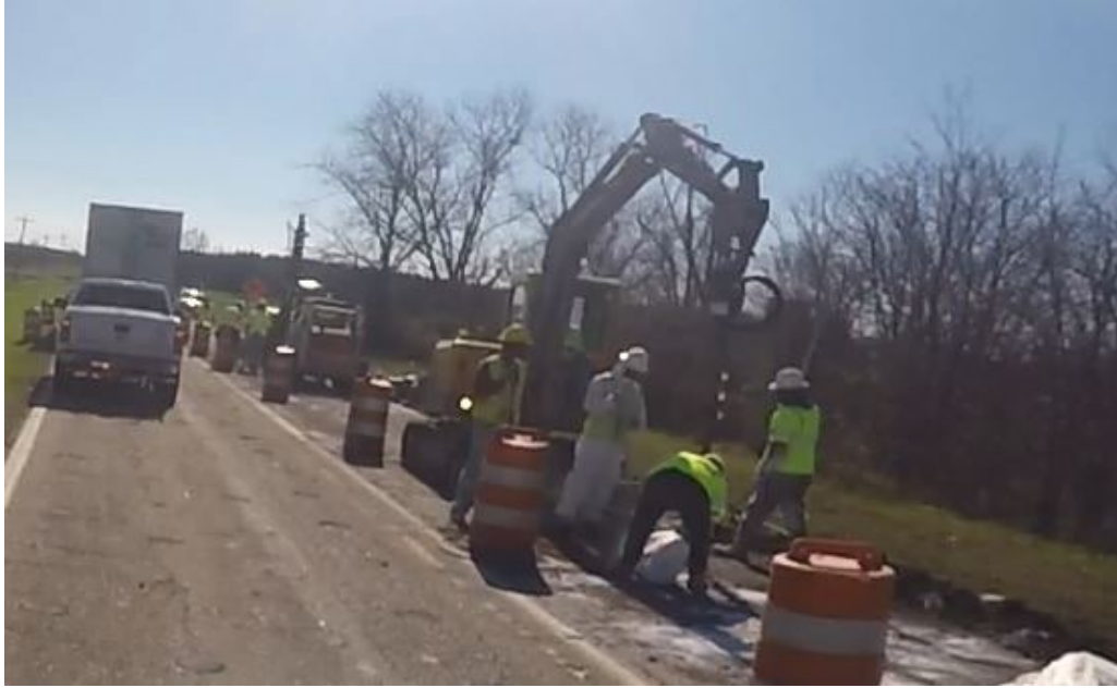
Figure 126: Packing Lime Columns
