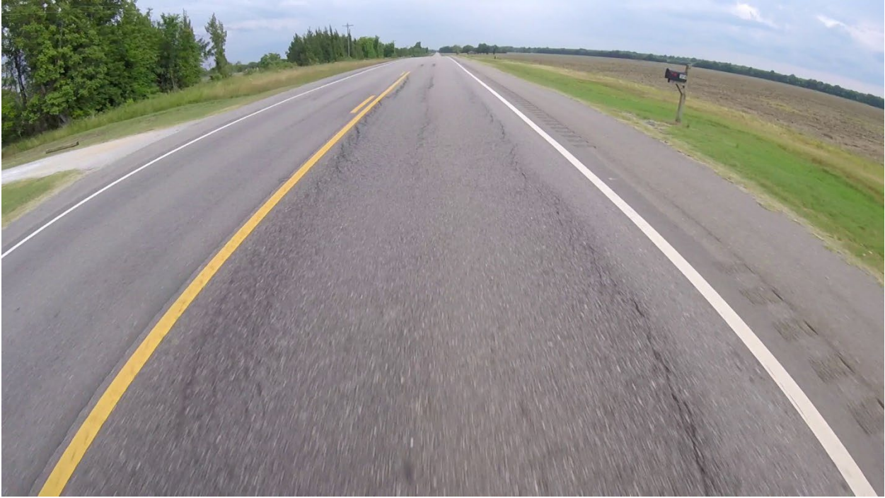
Figure 219: Shoving in Paved Shoulder Section
