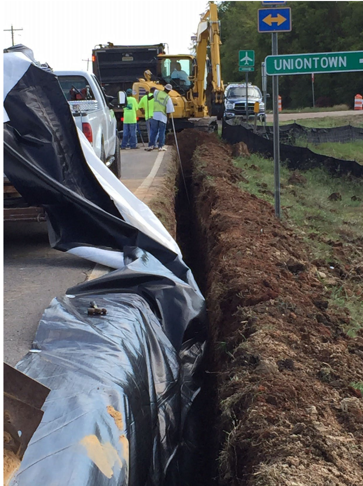
Figure 119: Vertical Moisture Barrier Membrane Placement
