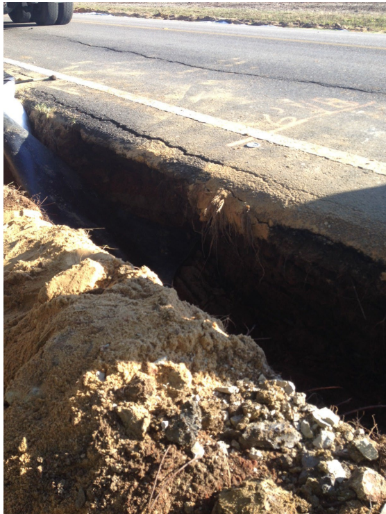
Figure 118: Vertical Moisture Barrier Cave-In
