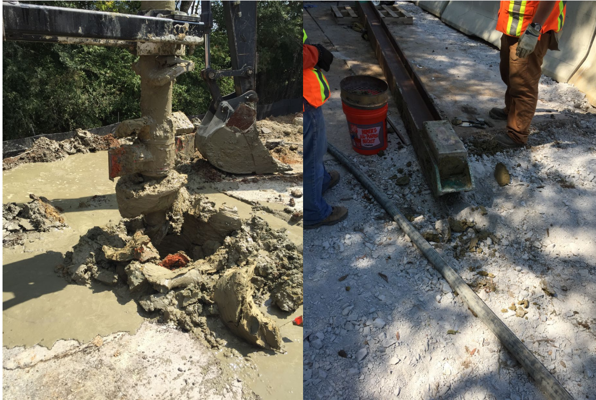
Figure 139: Deep Mix Columns Drilling and Sampling
