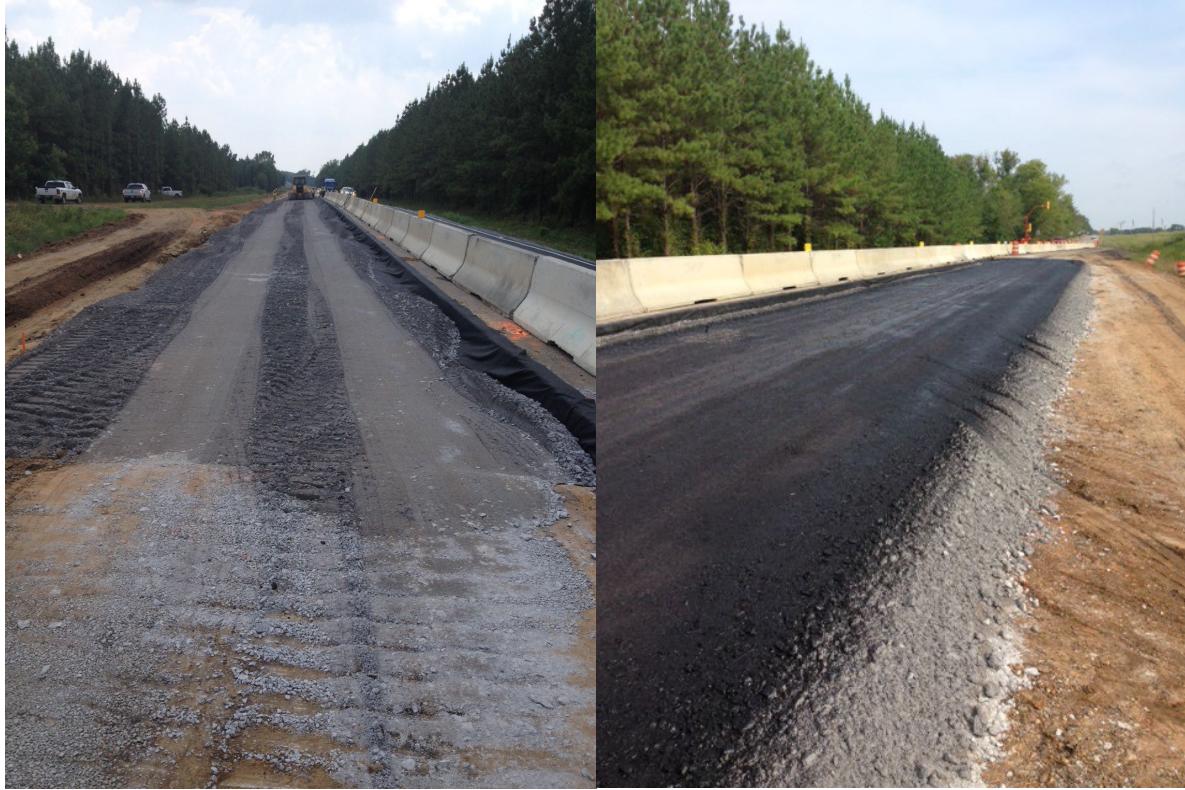
Figure 114: Sand Blanket Roadway Buildup
