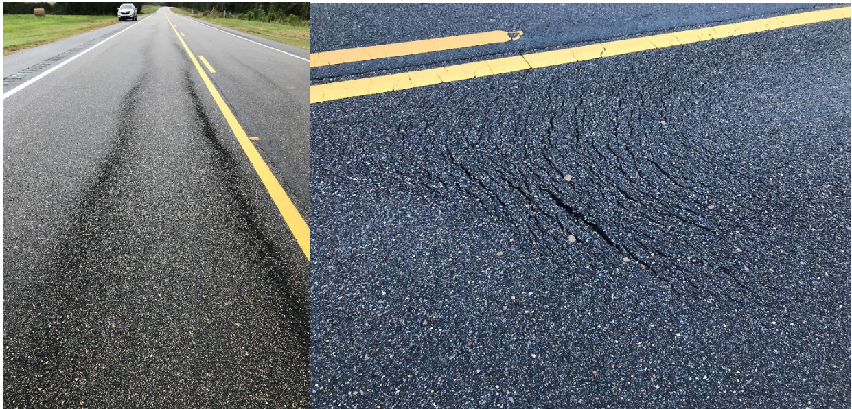
Figure 204: Visible Distress in paved shoulders section
