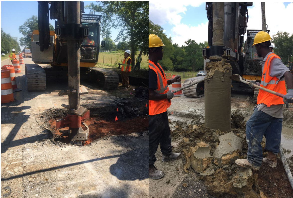
Figure 138: Deep Mix Columns Drilling
