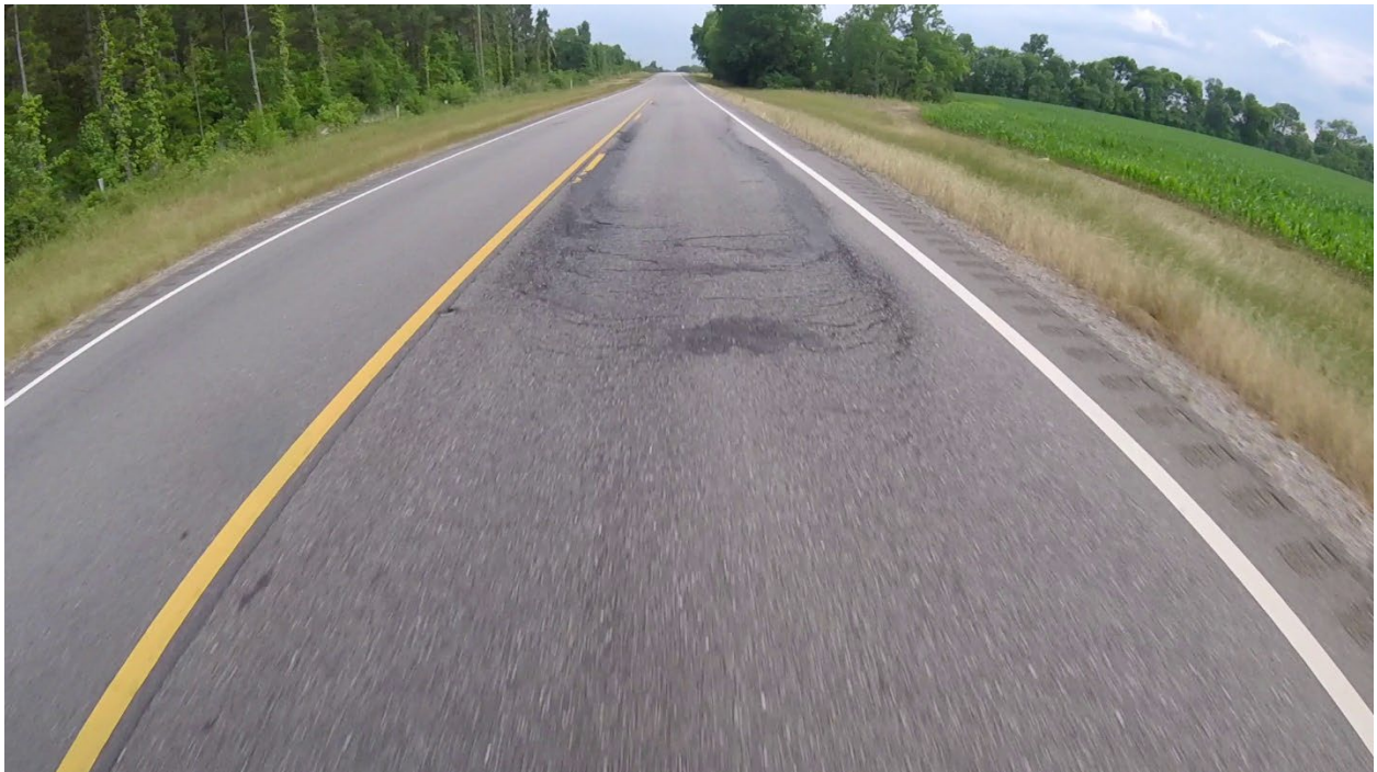
Figure 218: Shoving in Edge Drain Section
