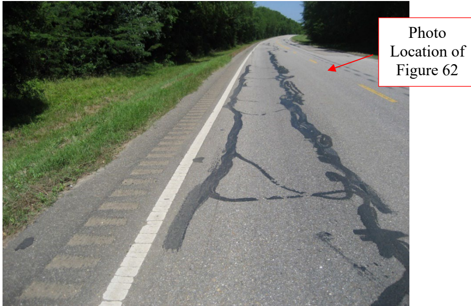
Figure 63: Observed Rutting and Longitudinal Cracking (Photo Taken 09/14/16)
