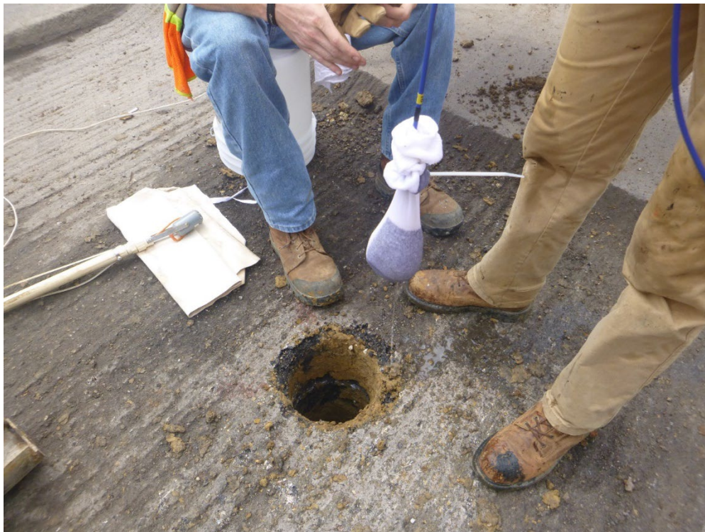
Figure 160: Piezometer in Sand-Filled Bag being Lowered Down the Borehole
