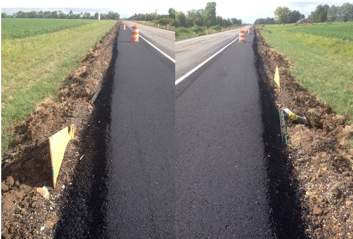
Figure 132: Paved Shoulder Build-Up
