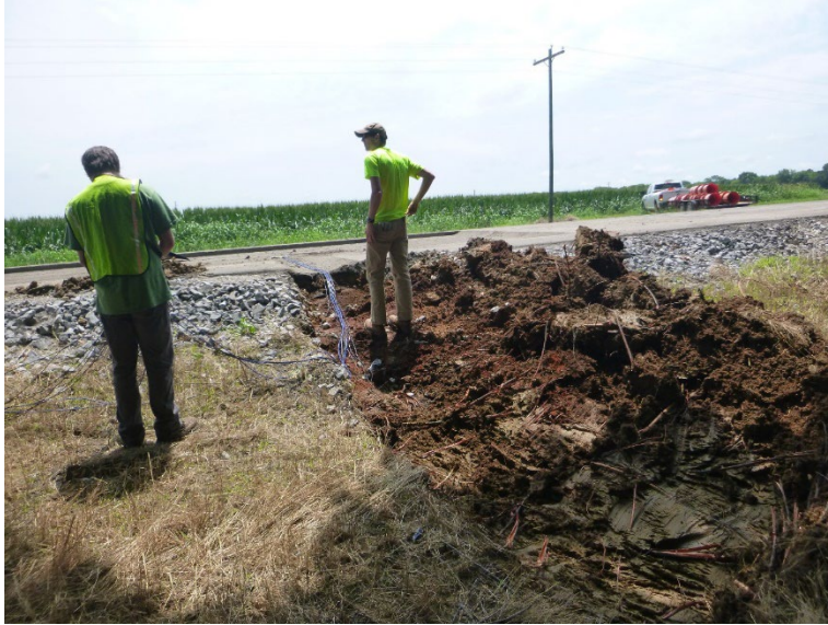
Figure 88: Tree Roots Observed During Installation of Sensors (Photo Taken 06/28/16)
