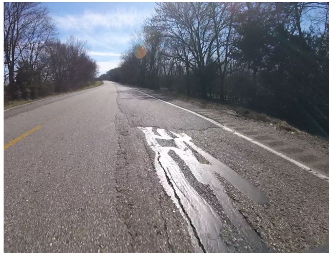
Figure 197: Longitudinal crack in Vertical Barrier section
