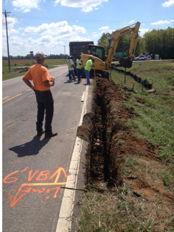
Figure 117: Vertical Moisture Barrier Excavation
