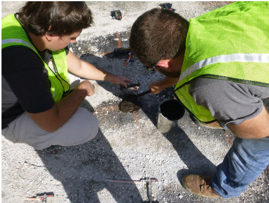
Figure 163: ASGs being Tacked with Tack-Sand Mixture
