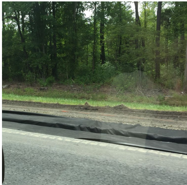
Figure 134: Edge Drain Excavation and Geotextile
