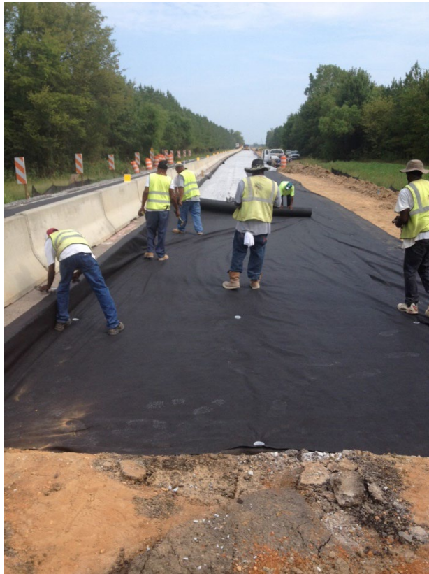
Figure 113: Sand Blanket Geosynthetic Layer
