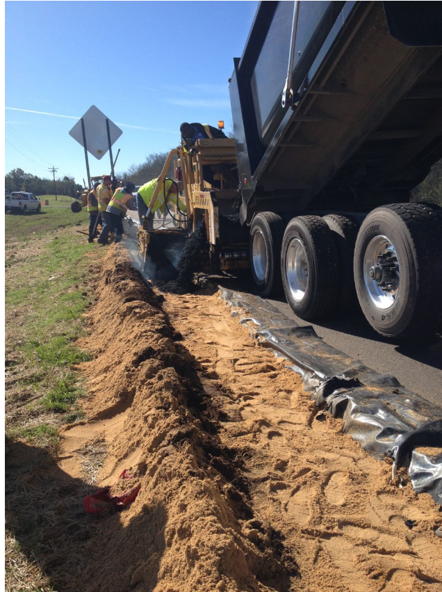
Figure 121: Vertical Moisture Barrier Paving
