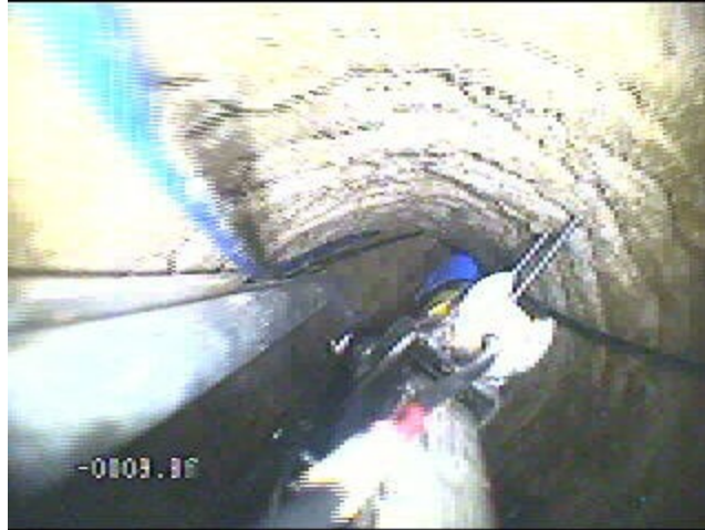
Figure 156: Moisture Sensor Installation
