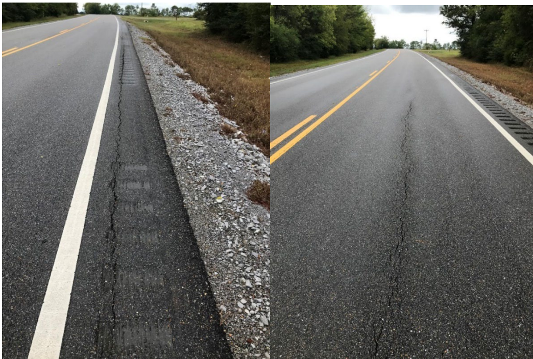
Figure 208: Shoulder and Lane Cracking in the Edge Drains
