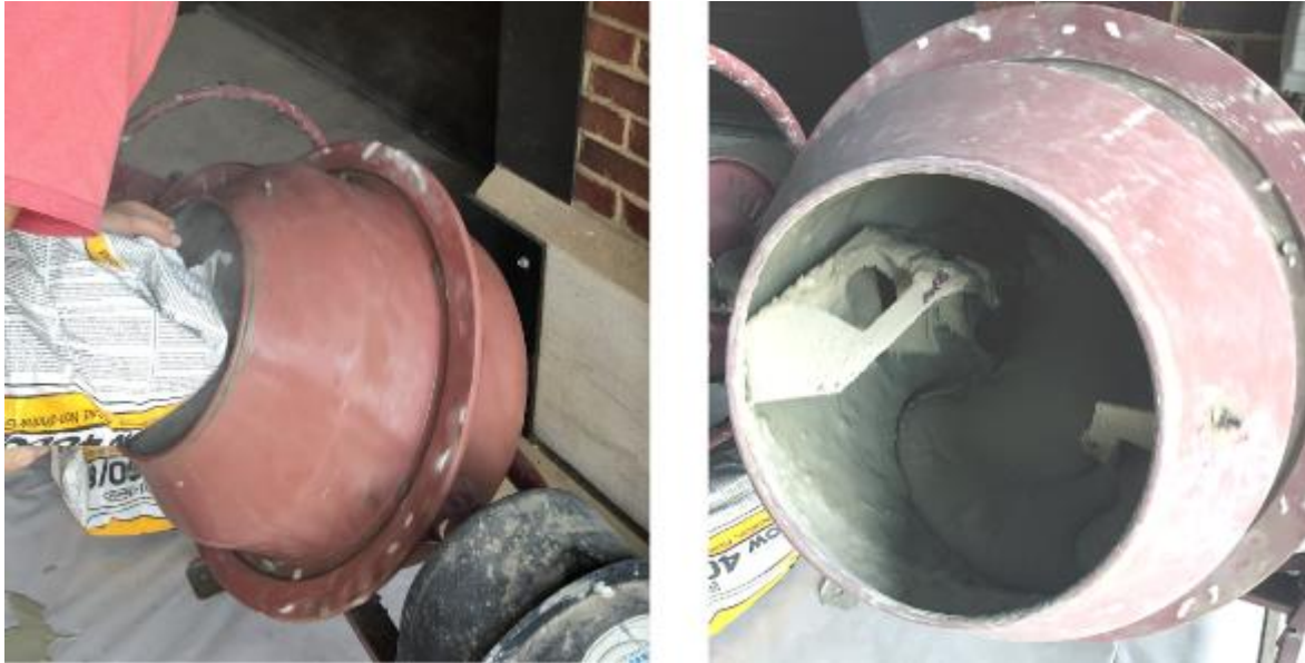
Figure 5-3 Figure showing grout preparation in a concrete mixer
