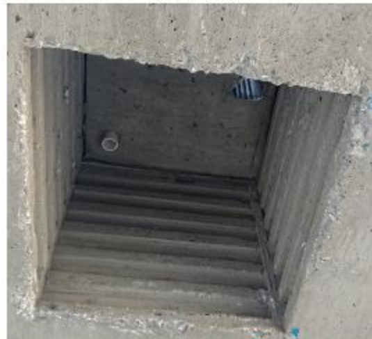
f) Interior of the void after casting
