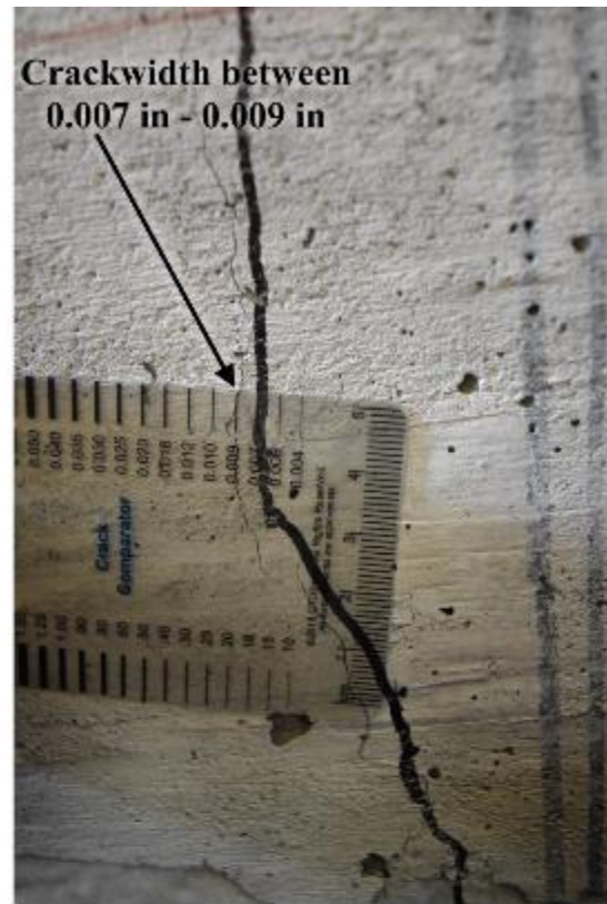
b) Closeup view showing crackwidth
