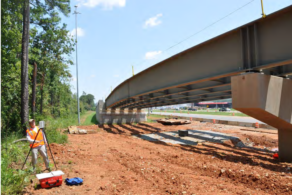
Figure 4.27: Scanner setup for Girder No. 1, erection condition
